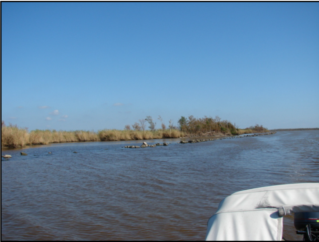
Photo No. 1, Typical rock dike
