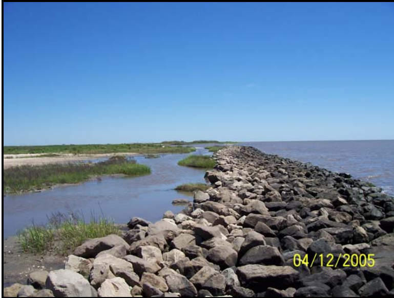
Photo 19. Area 4 Rock Dike – View of rock dike from end of Mobil Canal looking southeast, date: 4/12/05. Rock dike elevation appears to be very low.
