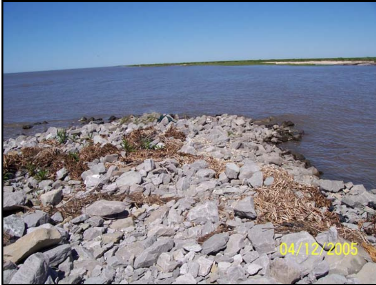
Photo 11. Plug No. 4A – View of west end of limestone rip rap plug looking west, date: 4/12/05
