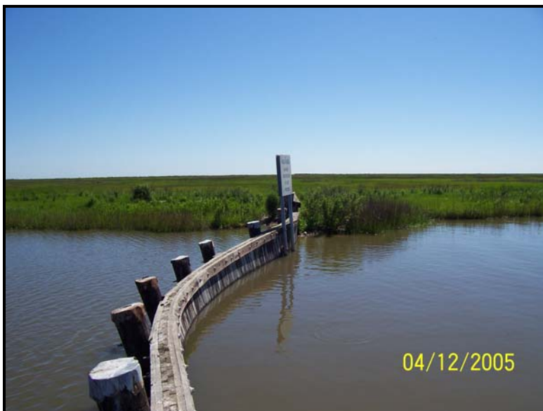
Photo 5. Plug No. 6 – View of plug deformation from centerline of plug looking east, date: 4/12/05
