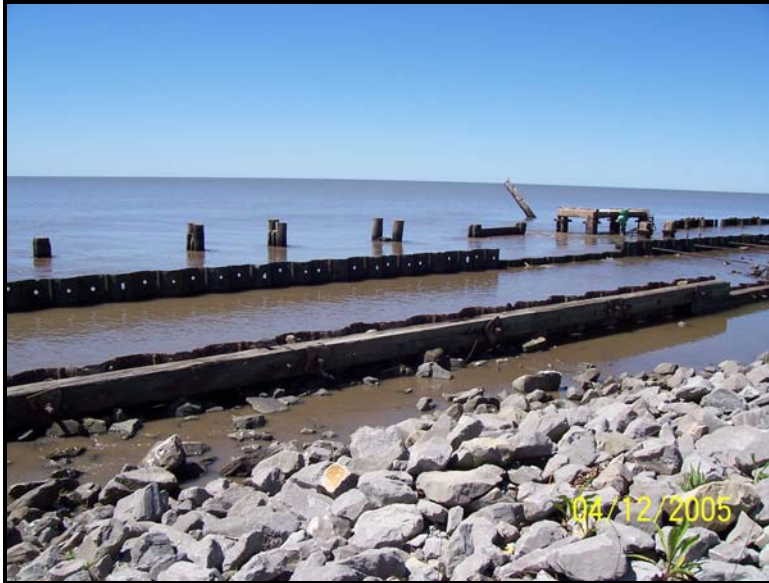
Photo 15. Plug No. 4A – View of bulkhead looking south, date: 4/12/05. Small breach just behind bulkhead where water is exchanging with Transco Canal at high tidal events. Also lower middle section of bulkhead can be seen where bulkhead is being overtopped in high tidal events.
