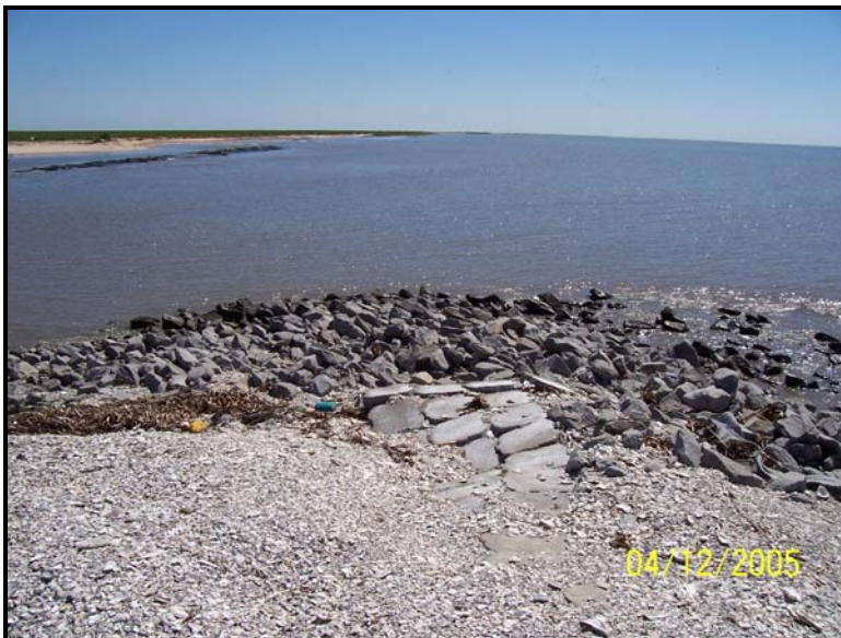
Photo 8. Plug No. 4A – View of east end of limestone rip rap plug looking east, date: 4/12/05.
