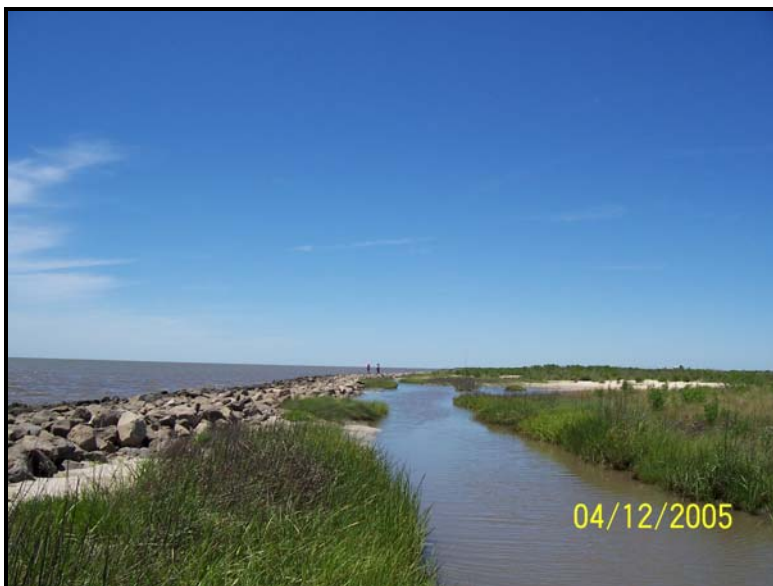
Photo 21. Area 4 Rock Dike – View of breach behind rock dike looking northwest, date: 4/12/05
