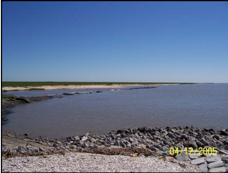
Photo 7. Plug No. 4A – View of east petraflex mats looking east, date: 4/12/05. Mats will be capped with limestone rip rap under TE-22 O&M Project.
