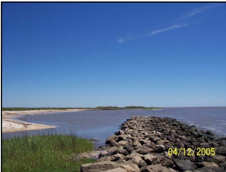
Photo 20. Area 4 Rock Dike – View of east end of rock dike looking southeast, date: 4/12/05. Adjacent shoreline is eroded approximately 50 – 75 feet behind rock dike.
