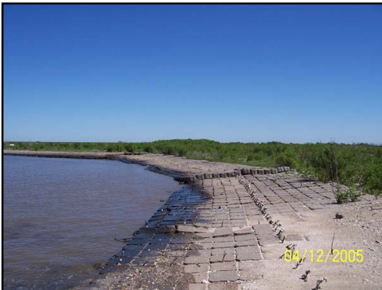
Photo 12. Plug No. 4A – View of west petraflex mats looking northwest, date: 4/12/05
