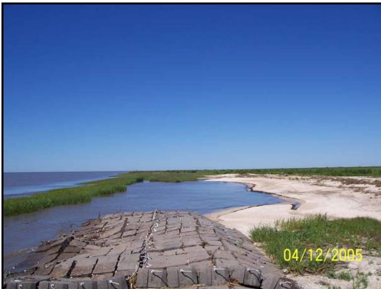
Photo 14. Plug No. 4A – View of the end of the west petraflex mats looking west, date: 4/12/05. Shoreline adjacent to mats is beginning to erode behind mats.
