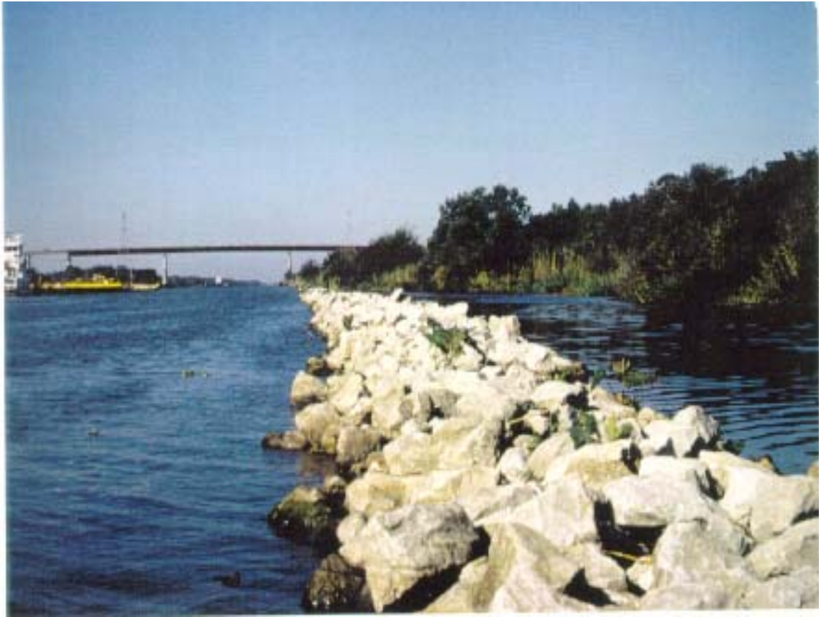
Figure 2. Photograph of the Cameron Prairie Refuge Protection (ME-09) project following construction in August 1994, illustrating the shoreline of the GIWW and the installed rock breakwater.
