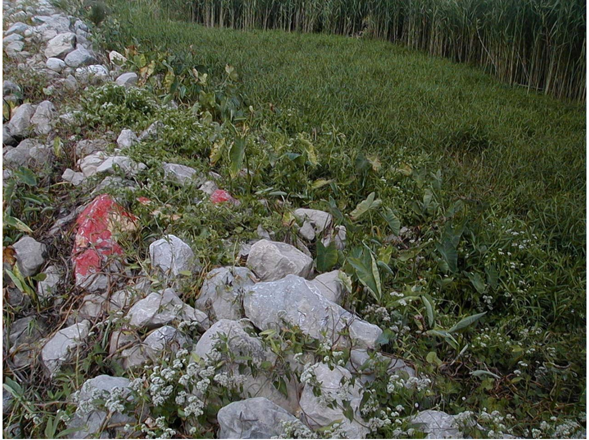
Figure 7. View of the Cameron Prairie rock dike showing naturalized vegetation colonizing the dike itself and the accreted marsh behind the dike. The red paint was used to mark the location of the shoreline marker for the DGPS survey.
