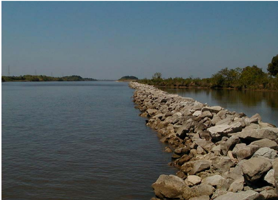
Photo 2—typical section of dike (April, 2005)
