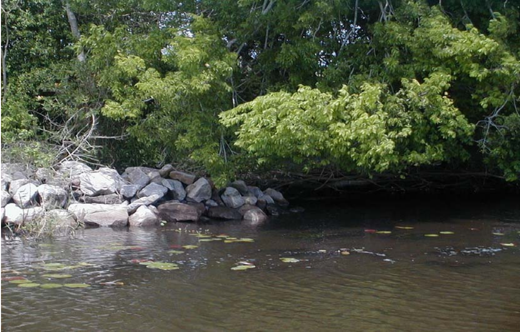
Photo 1—southern tie-in on the Burton-Sutton Canal
