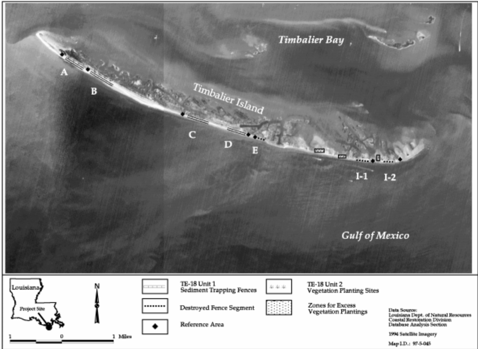
Figure 1. Timbalier Island Plantings (TE-18) project elements. Letters (A-I) represent fence segments.
