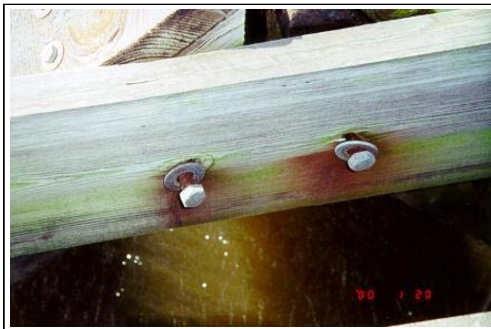
Figure 24. Typical structural damage exhibited by the Grated Apex and Angled Timber Fence structures at the Lake Salvador Shoreline Protection (BA-15) Demonstration project (photo taken January 2000).
