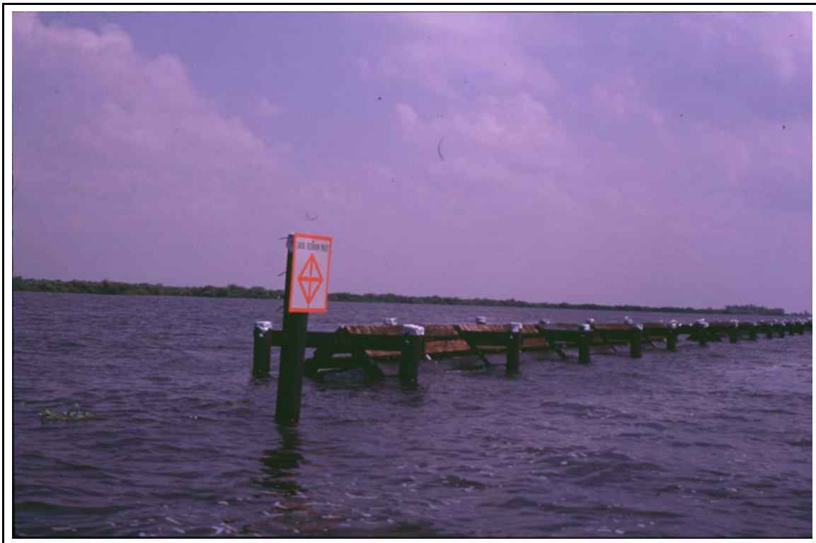
Figure 6. Typical Grated Apex structure at the Lake Salvador Shoreline Protection (BA-15) Demonstration project (photo taken December 1998).
