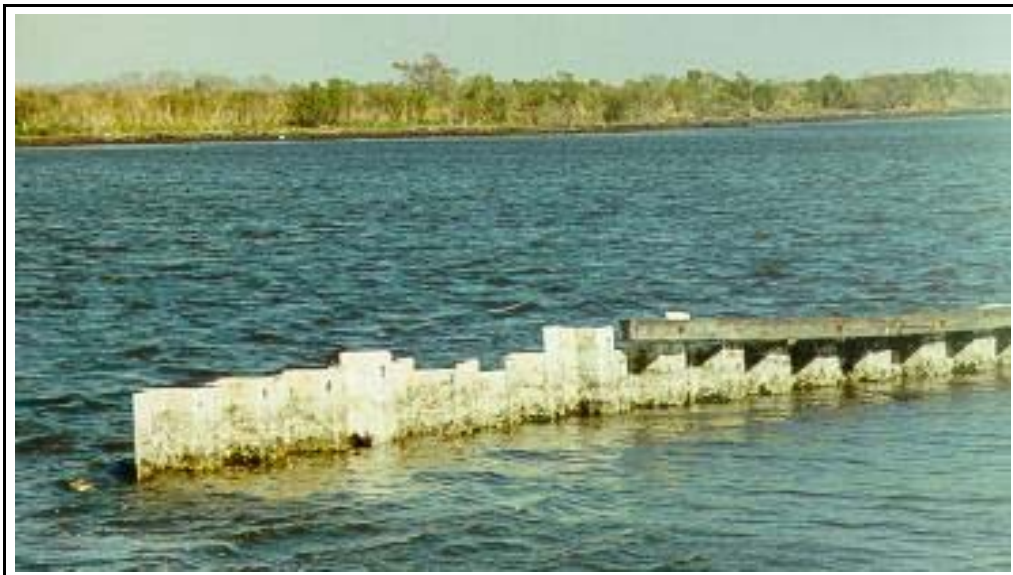
Figure 22. Typical structural damage to the unreinforced Vinyl Sheet Pile structures at the Lake Salvador Shoreline Protection (BA-15) Demonstration project (photo taken January 2000).
