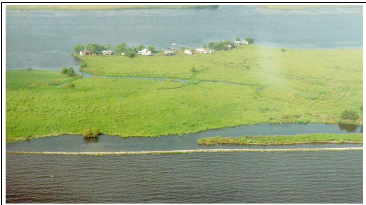
Figure 10. Typical Geotextile Tube structure at the Lake Salvador Shoreline Protection (BA-15) Demonstration project (photo taken August 1998).
