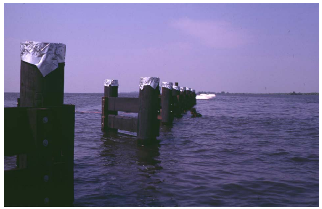
Figure 8. Typical Angled Timber Fence structure at the Lake Salvador Shoreline Protection (BA-15) Demonstration project (photo taken December 1998).
