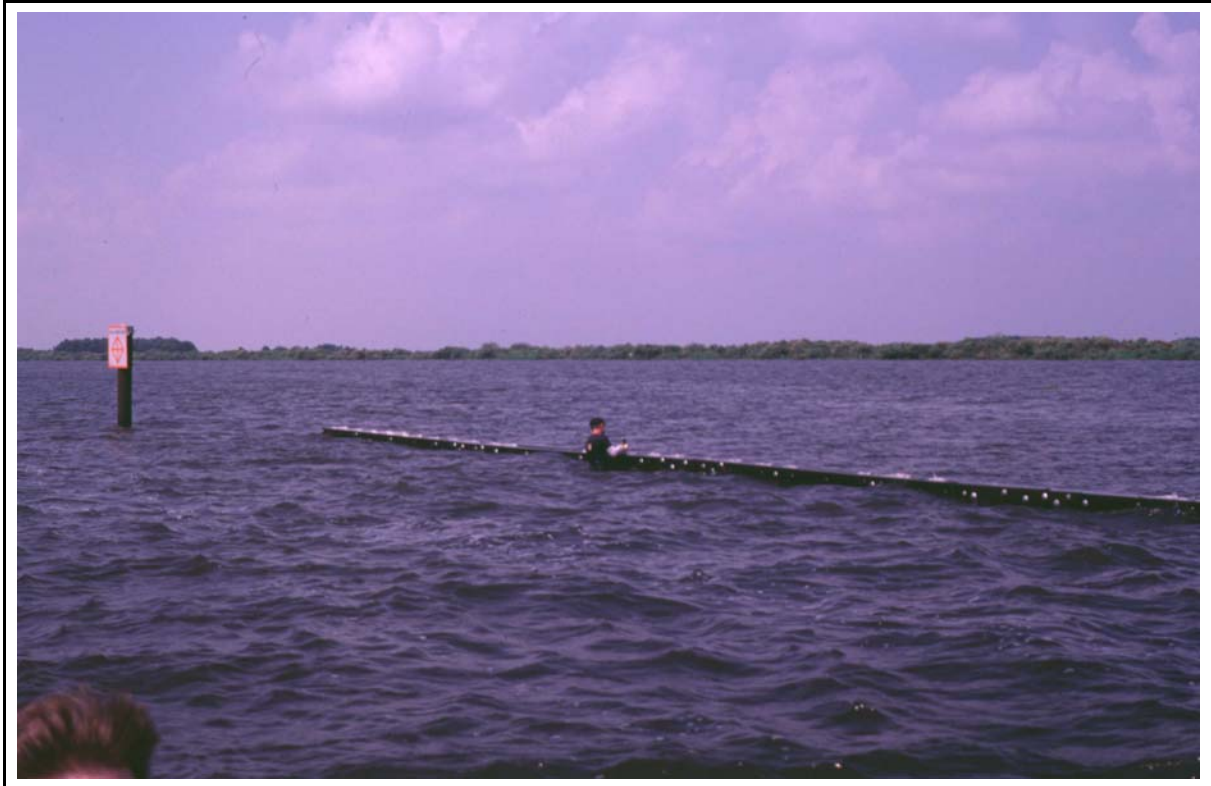
Figure 9. Typical Vinyl Sheet Pile structure at the Lake Salvador Shoreline Protection (BA-15) Demonstration project (photo taken in December 1998).
