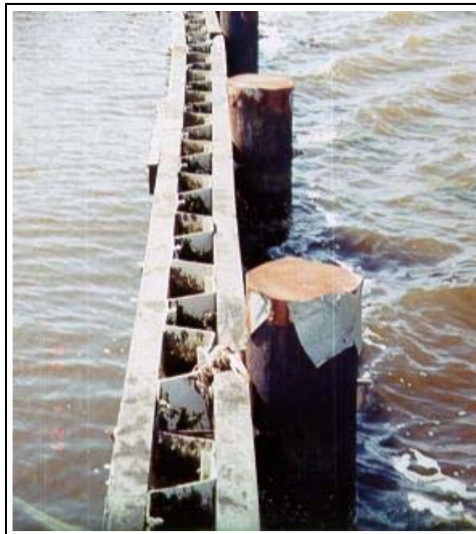
Figure 23. Typical structural stability of the reinforced Vinyl Sheet Pile structures at the Lake Salvador Shoreline Protection (BA-15) Demonstration project (photo taken January 2000).
