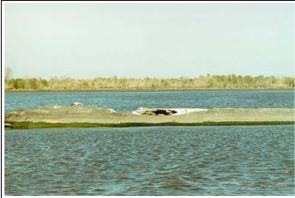
Figure 21. Typical damage to the Geotextile Tube structures at the Lake Salvador Shoreline Protection (BA-15) Demonstration project (photo taken January 2000).
