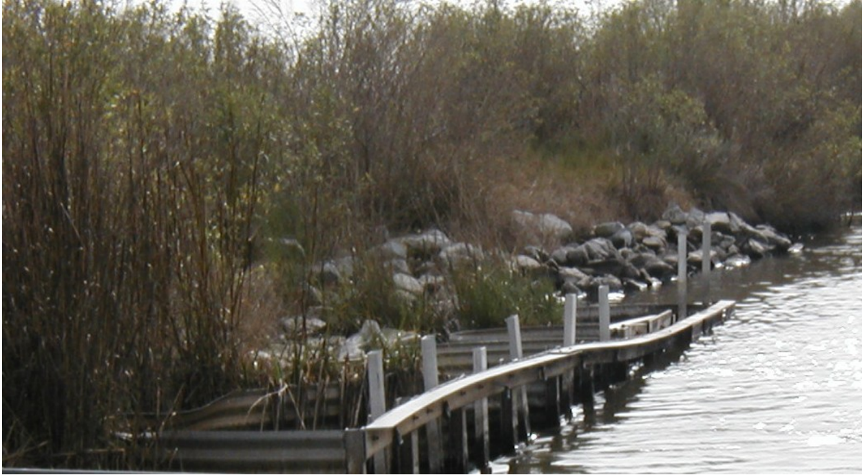
Figure 4 East Mud Lake (CS-20) structure 4 showing sinkage of the southern end.
