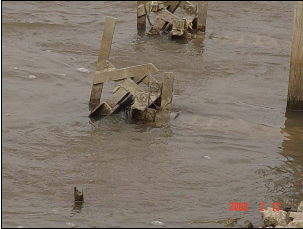
Photo 3, Outlet side of Structure No. 1.
