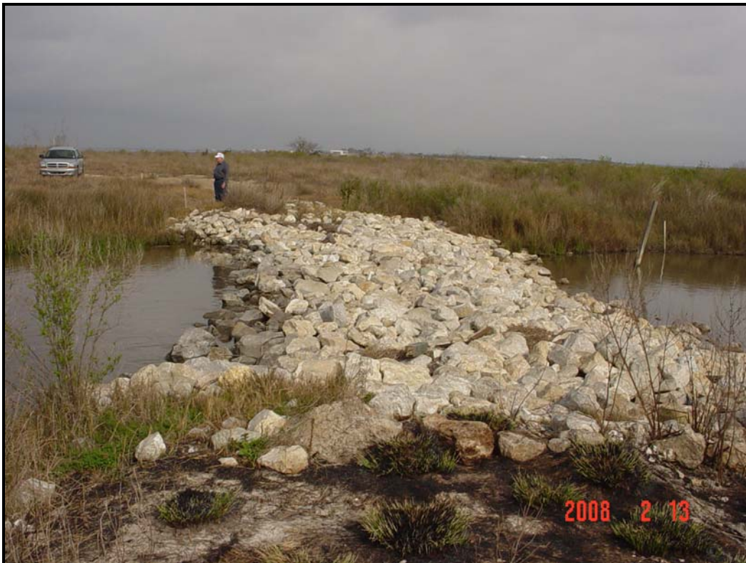
Photo 8, Rock plug at structure No. 8.
