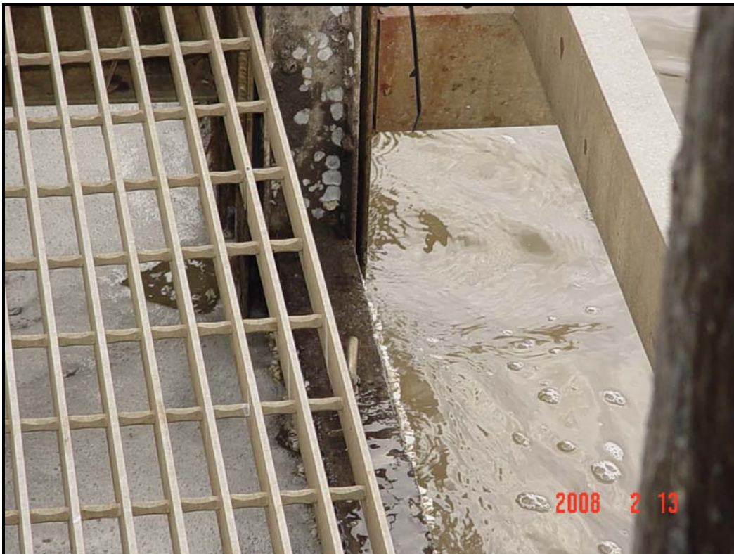
Photo 4, Inlet side of Structure No. 12.
