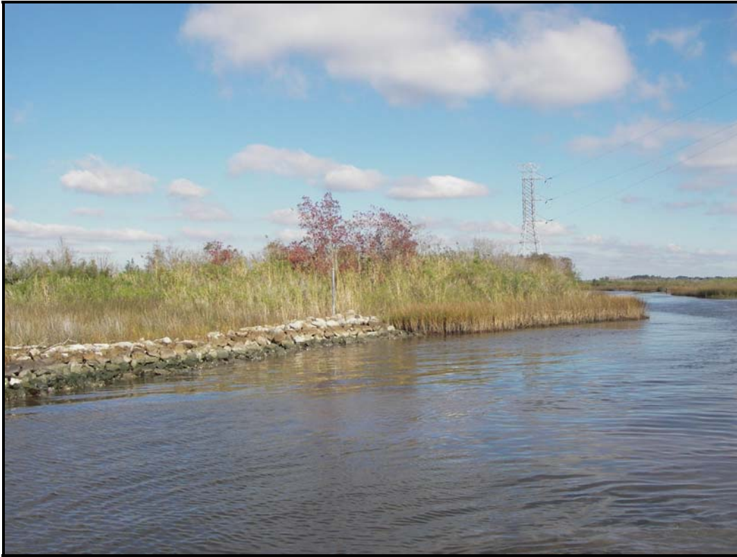
Photo 1 —East tie-in at Alkali Ditch.
