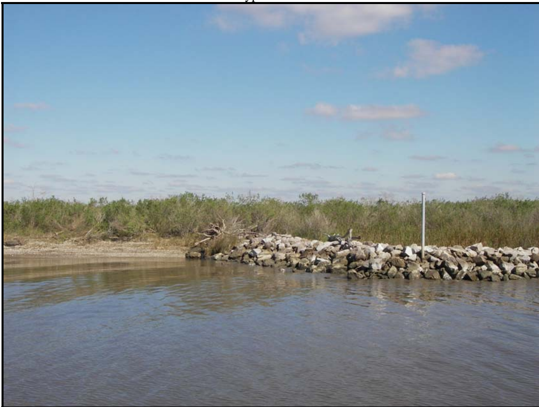
Photo 4 —Western tie-in of dike.
