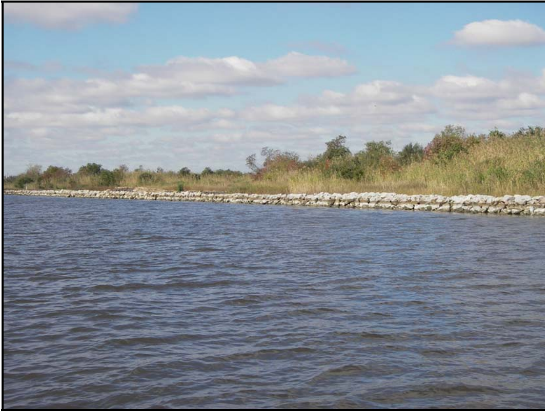
Photo 3 —Typical section of dike.
