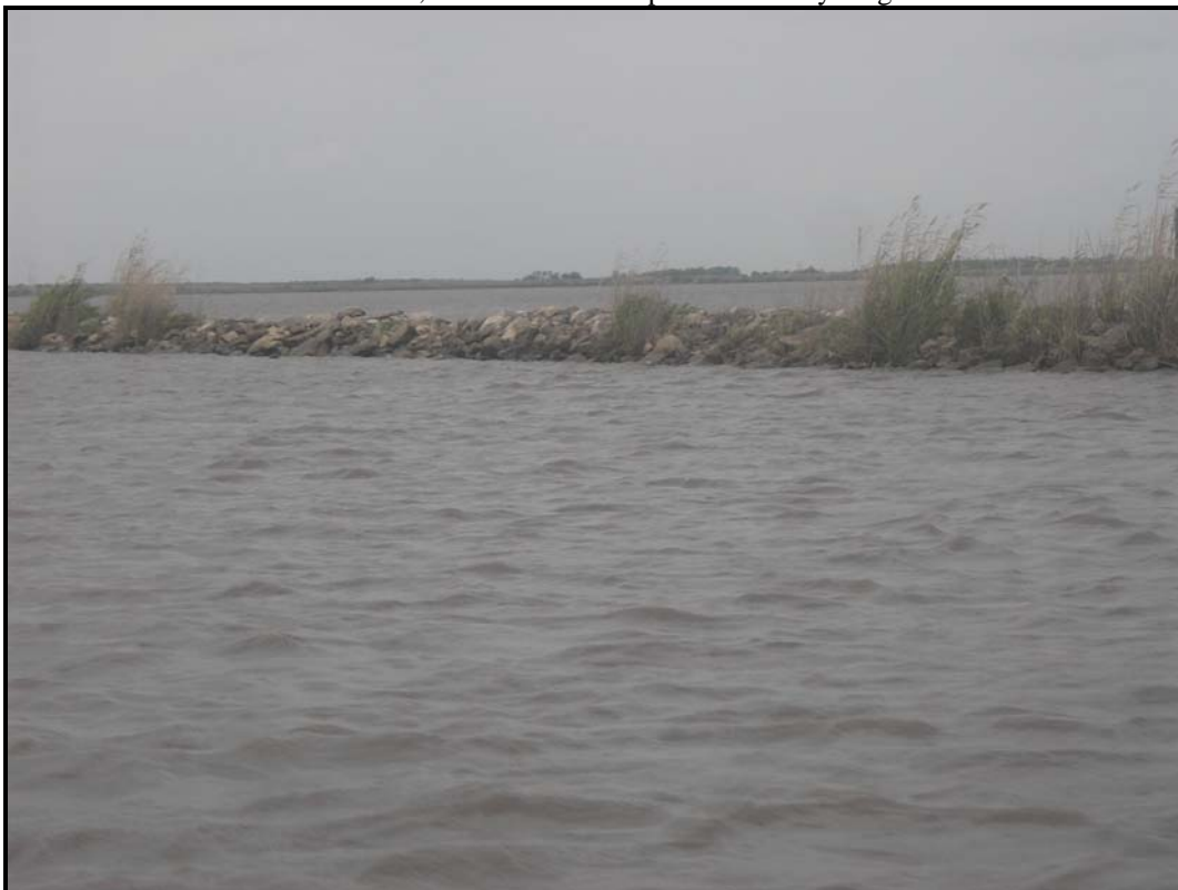
Photo No.2 , Typical rock dike section.
