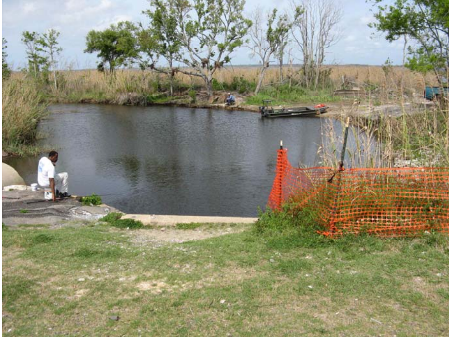
Photo #1 –Salt Bayou Scour. Facing the north bank of Salt Bayou inside the project area from the Hwy 90 culverts. Note the large section of bank which has been scoured out.
