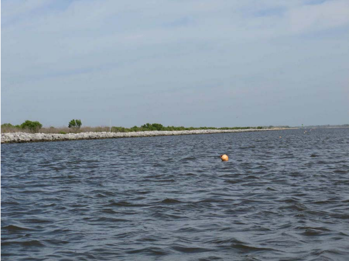
Picture 2. Shoreline protection.
