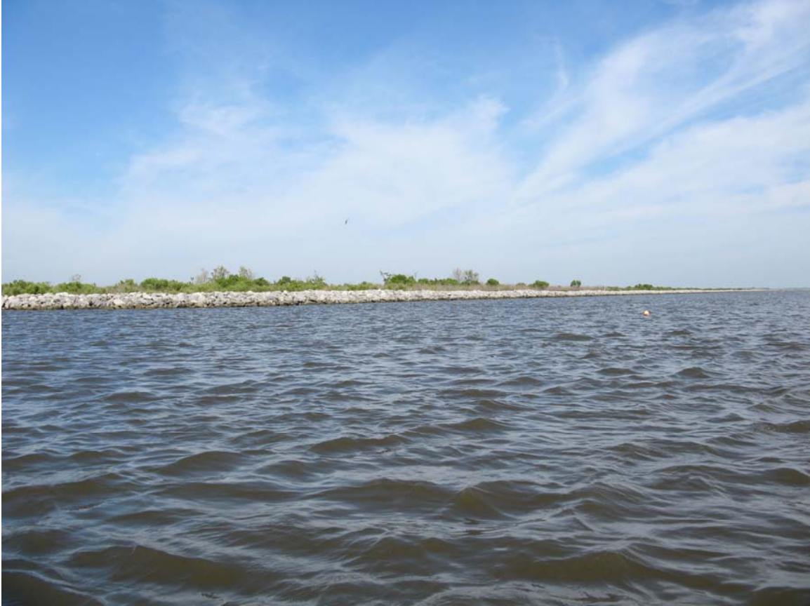
Picture 1. Shoreline protection.
