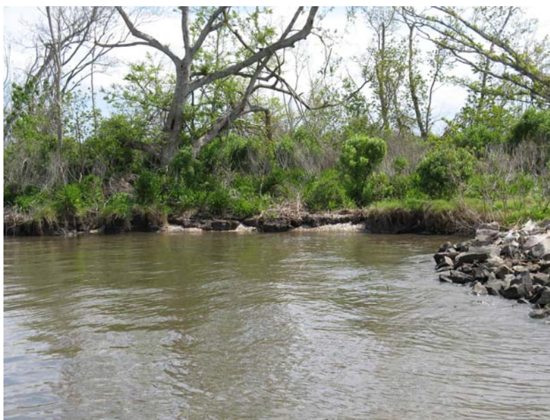
Photo 11 Bank erosion at west end of Bayou Perot Rock Dike
