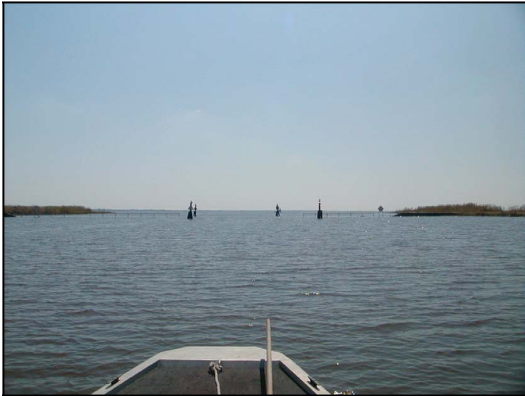
Photo 5 —missing sign and Nav-Aid lights at Humble Canal
