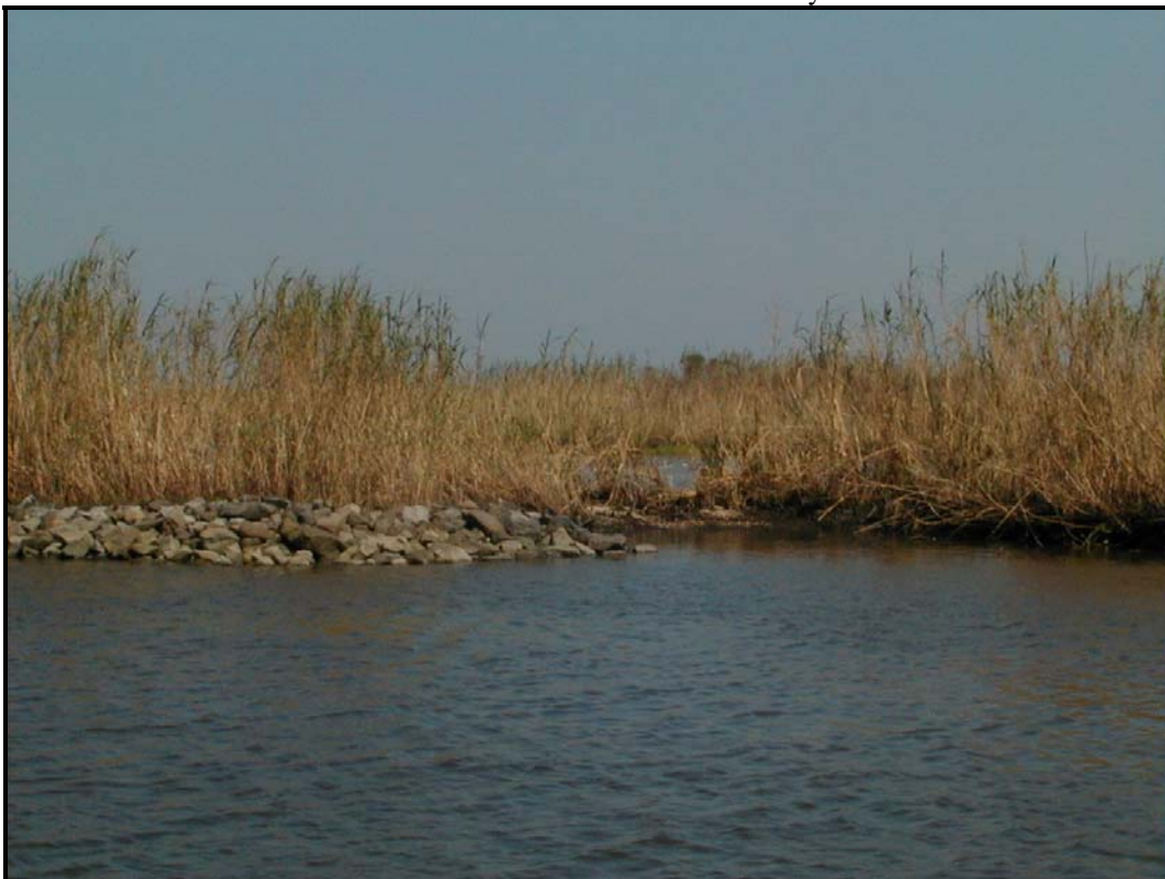
Photo 8 — south end of rock dike at location closure near Humble Canal
