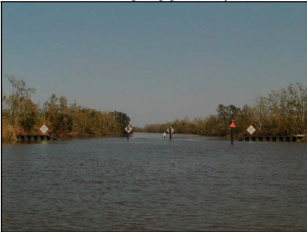
Photo 12 —British American Canal structure and signage
