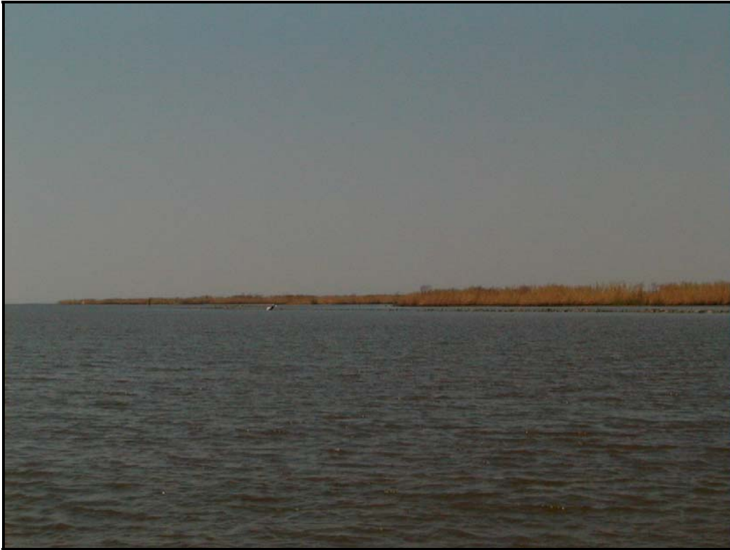
Photo 9 —typical section of School Bus dike
