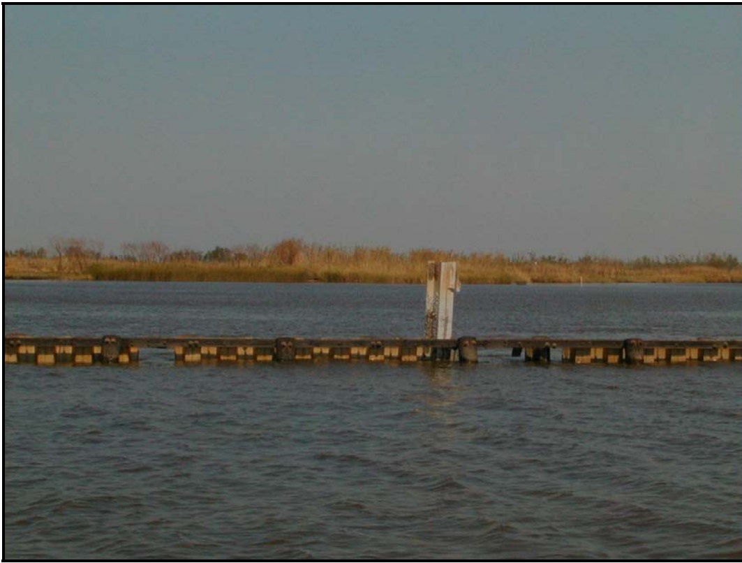
Photo 15 —typical section of PVC wall
