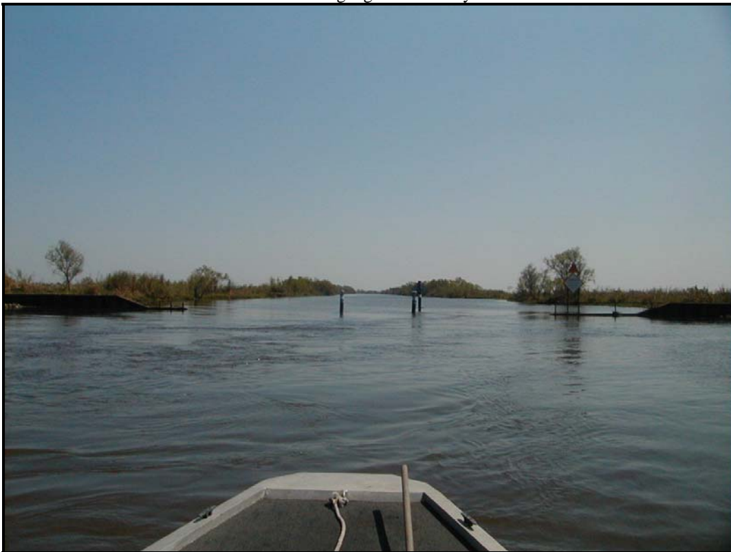
Photo 2 — Missing sign, nav-aid marker, and railing @ Humble F Canal (on left)
