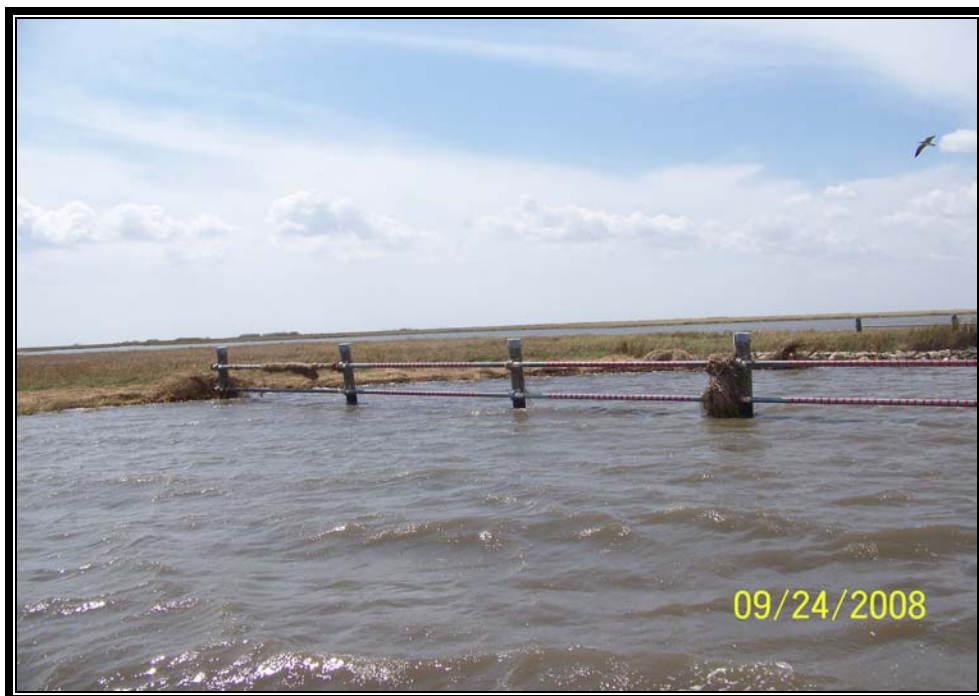
Photo No. 12 – view of the rock weir tie-in to the existing marsh and barricade system on the south side of Structure No.4
