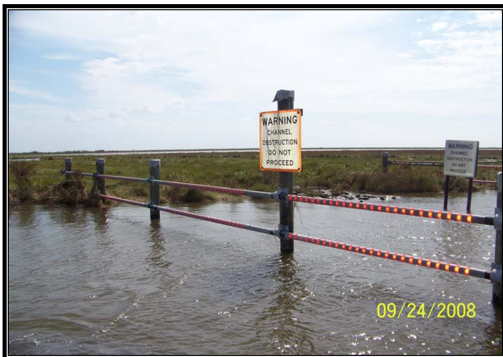
Photo No.14 – rock weir tie-in to marsh and barricade system on the north side of Structure No.5.
