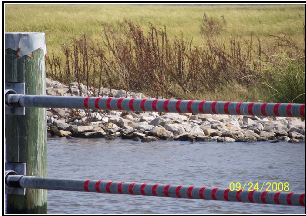
Photo No.23 – barricade system and rock weir tie-in along the west bank of Structure No.9.
