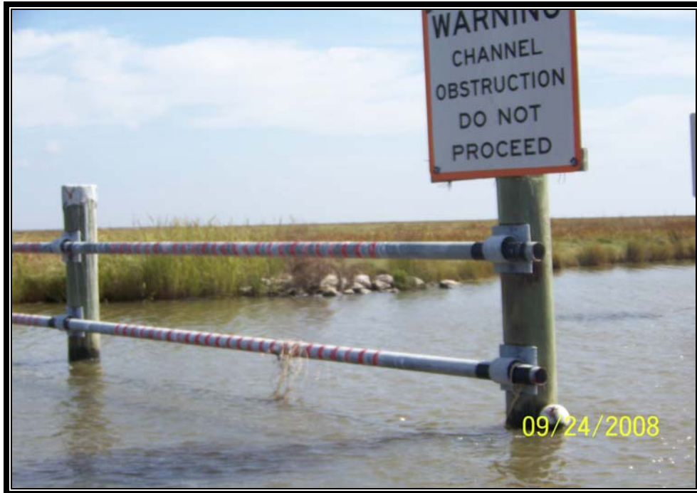
Photo No. 17 – rock weir tie-in to marsh and barricade system on the north side of Structure No.6.
