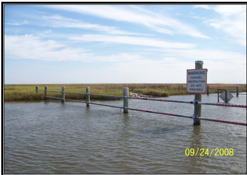
Photo No. 20 – barricade system and rock weir tie-in to marsh on the north side of Structure No.7.
