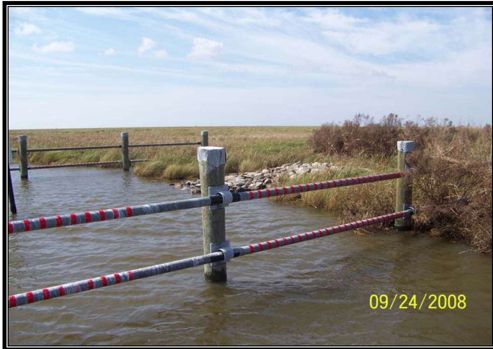
Photo No. 13 – rock weir tie-in to marsh and barricade system on the south side of Structure No.5.
