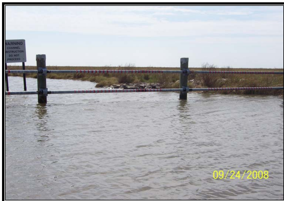
Photo No. 16 – rock weir tie-in to marsh and barricade system on the south side of Structure No.6.
