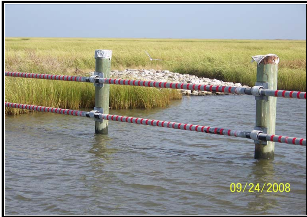
Photo No.3 – view of the barricade system and rock weir tie-in on the west side of Structure No.1
