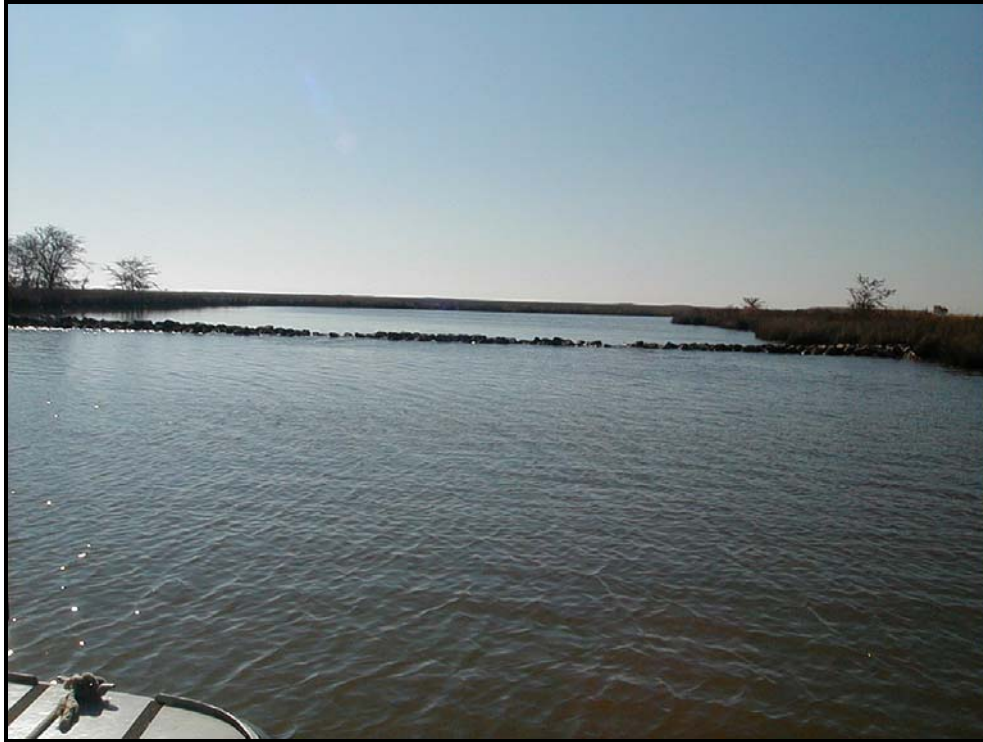
Photo 1, Closure No. 1. Note low areas of stone in center of structure.
