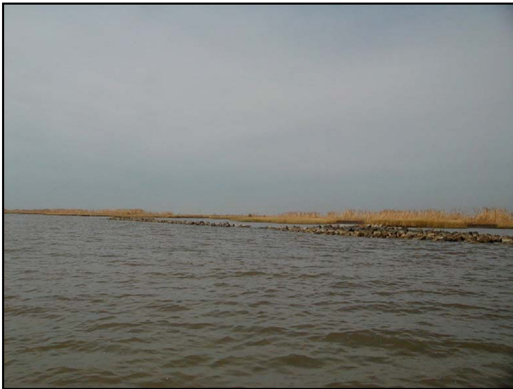
Photo 10, Closure No. 9, along south shore of Marsh Island. Note that shoreline protection dike is now away from the current shoreline post-Hurricane Rita.
