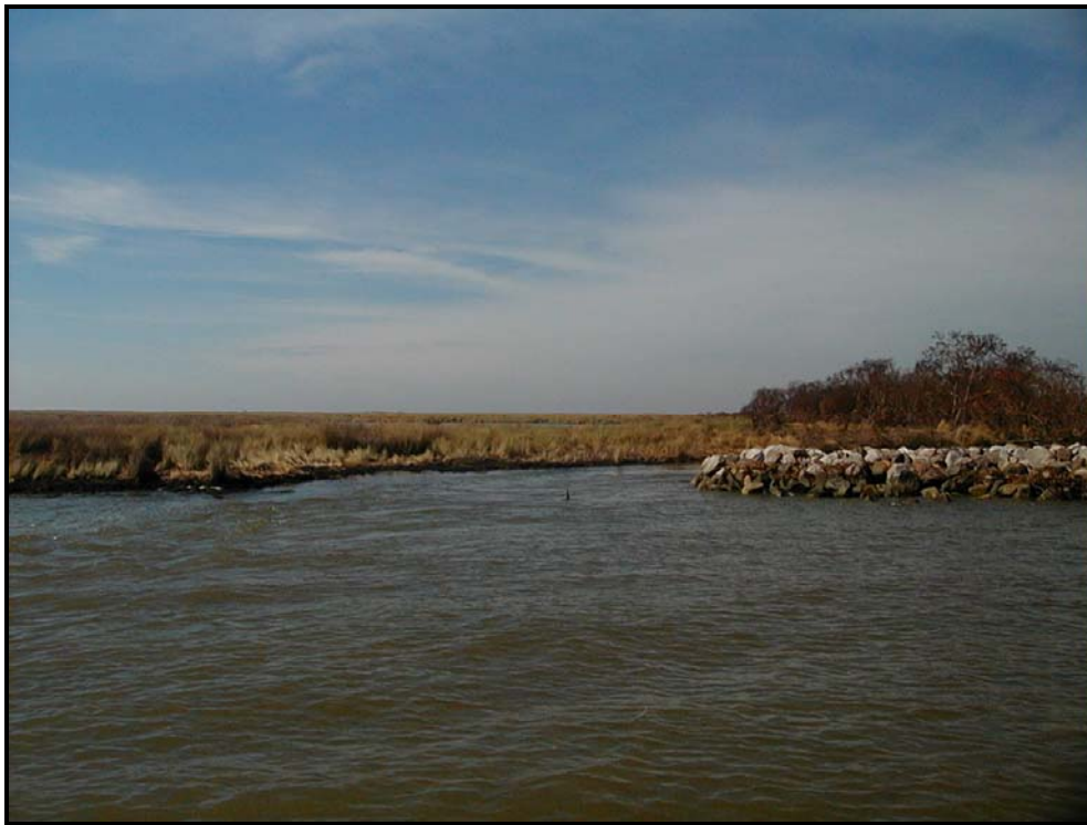
Photo 7, Closure No. 6. Note breach on south end of closure stone fill. Breach had begun prior to Hurricane Rita but was not as wide.
