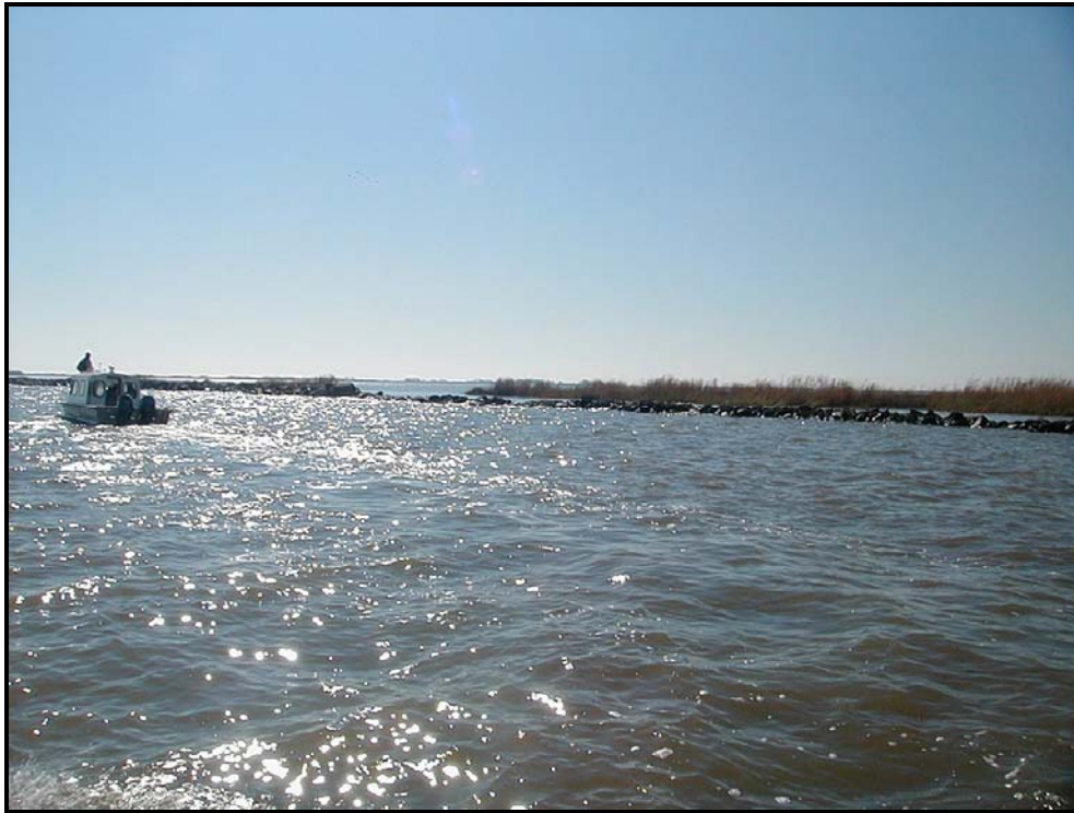
Photo 5, East end of Lake Sand Closure No. 4. Note low areas of stone.
