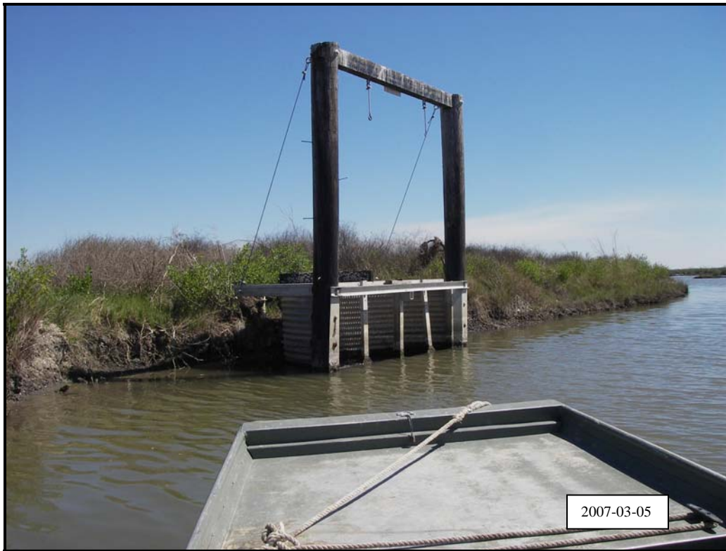
Photo 9, Structure No. 11, view showing erosion either side of structure.
