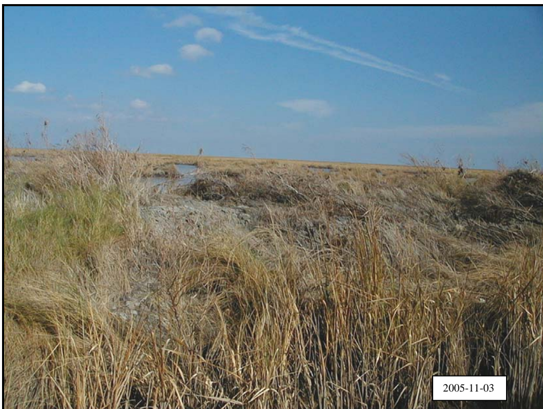
Photo 21, North Levee, looking east, showing washout of top portion of levee.
