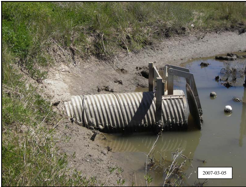
Photo 15, Structure No. 3, showing outlet pipe and flap gate.
