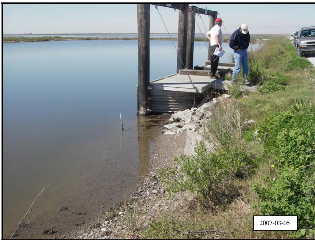
Photo 5, Structure No. 8, view looking southwest, showing bank line erosion.
