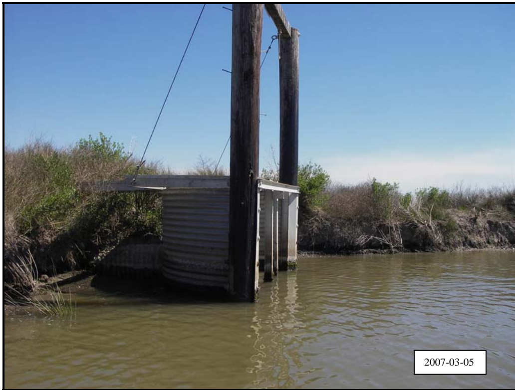
Photo 11, Structure No. 5, showing erosion either side of structure.
