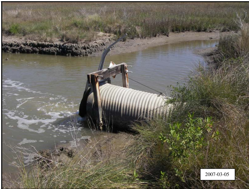
Photo 12, Structure No. 5, showing outlet pipe and flap gate with missing boardwalk.
