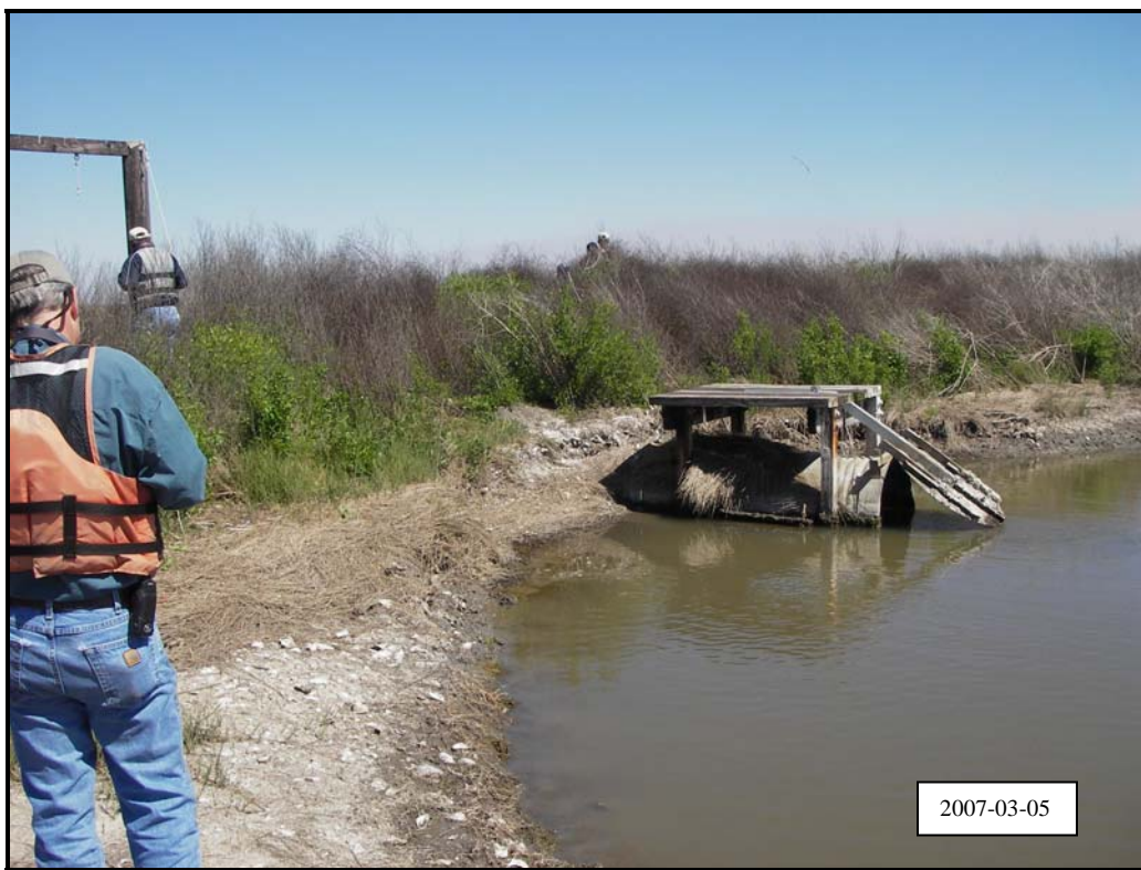
Photo 17, Structure No. 1, showing outlet pipe flap gate and erosion around structure.
