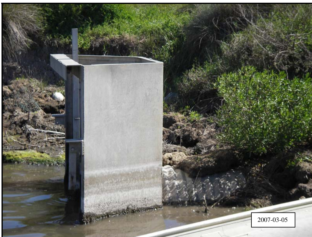
Photo 14, Structure No. 3, showing erosion and missing boardwalk.
