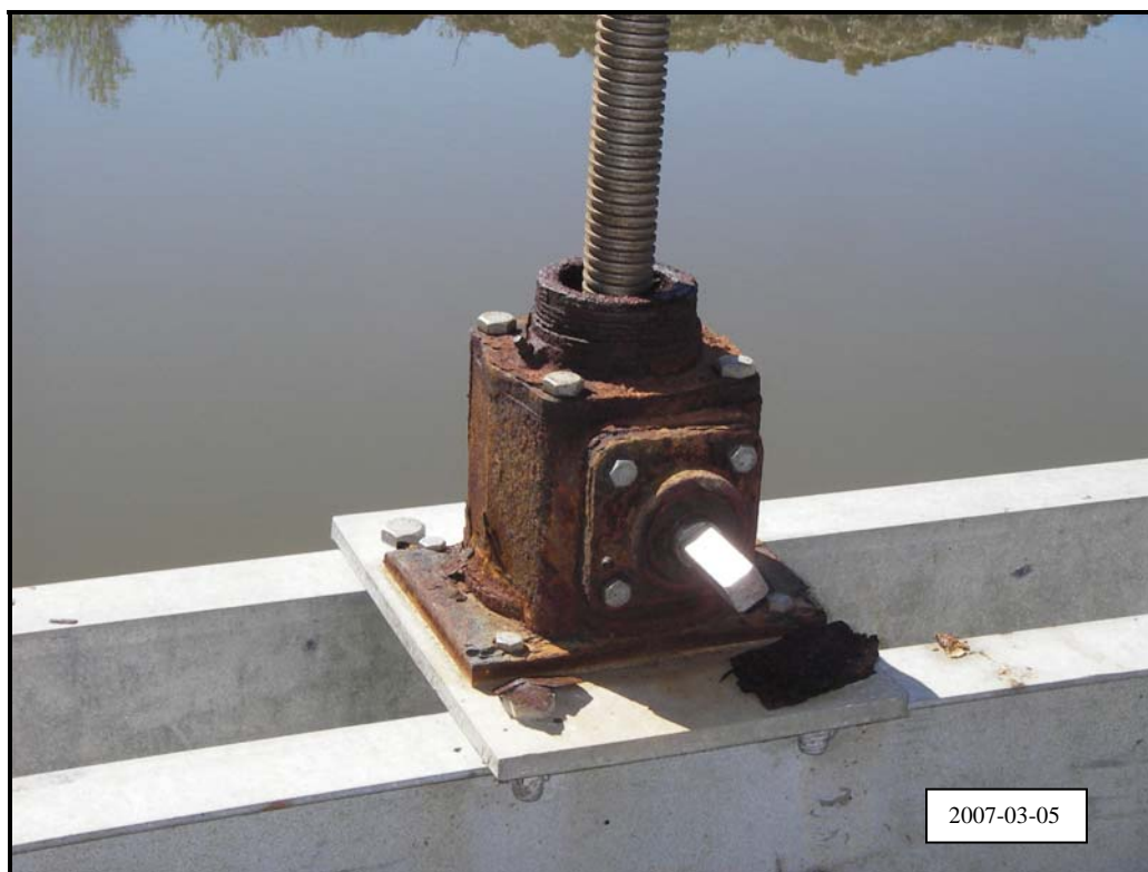
Photo 8, Structure No. 9b, showing corrosion on gear box & missing stem cover.
