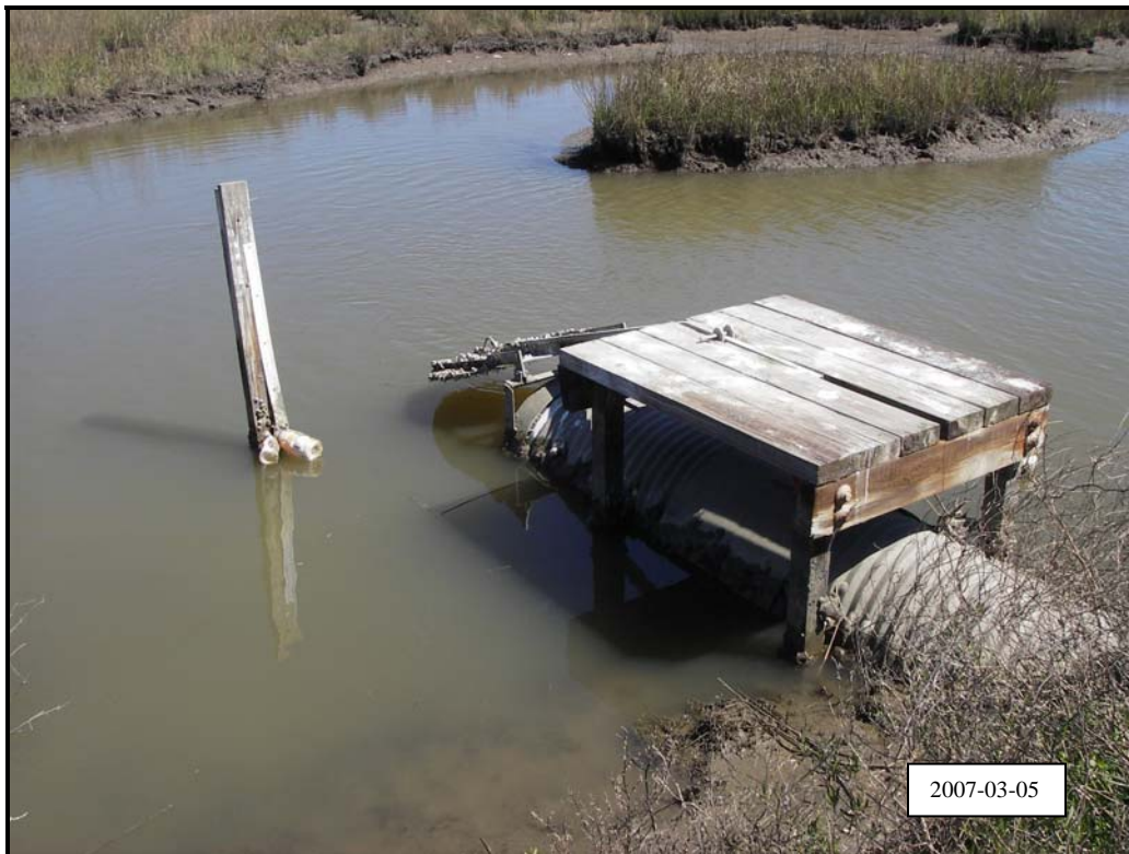
Photo 10, Structure No. 11, outlet pipe and flap gate.
