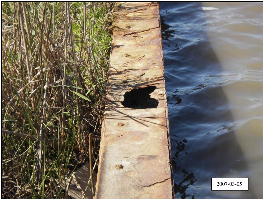
Photo 20, Structure No. 13, showing corrosion on sheet pile cap.
