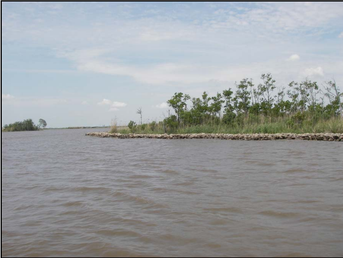
Photo No. 1 , typical section of dike
