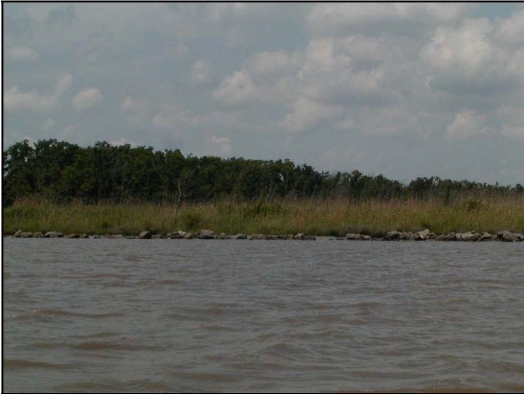
Photo 1, Typical rock dike
