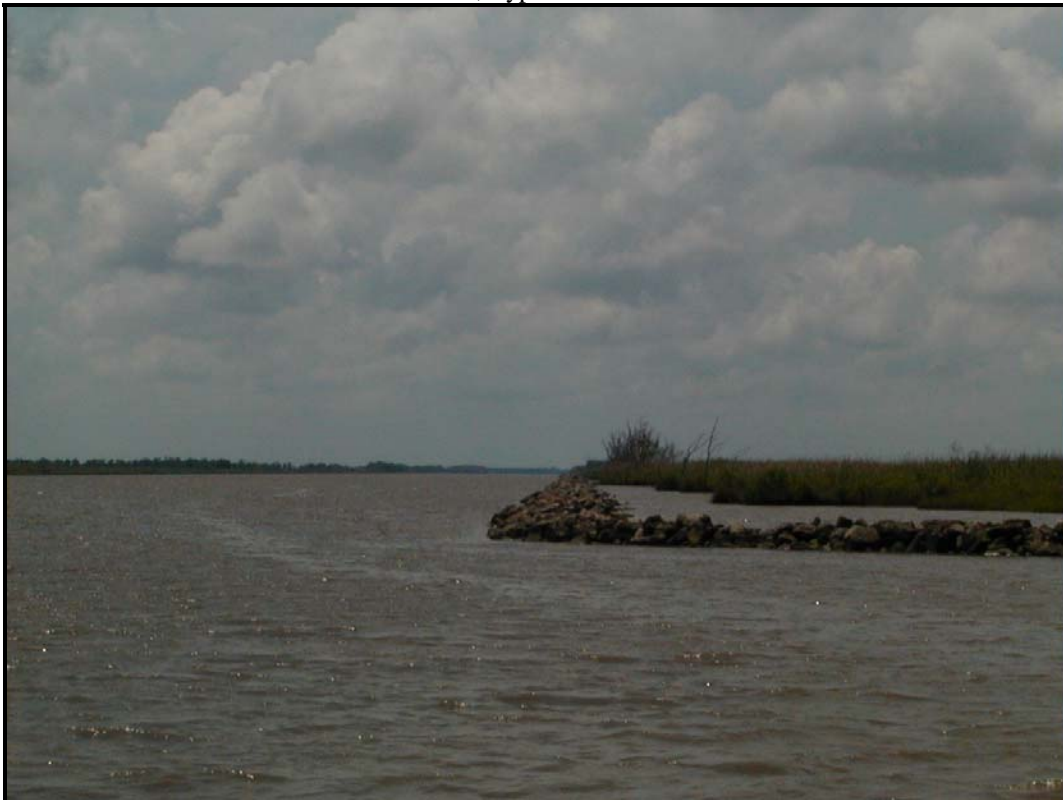
Photo 2, Typical rock dike.
