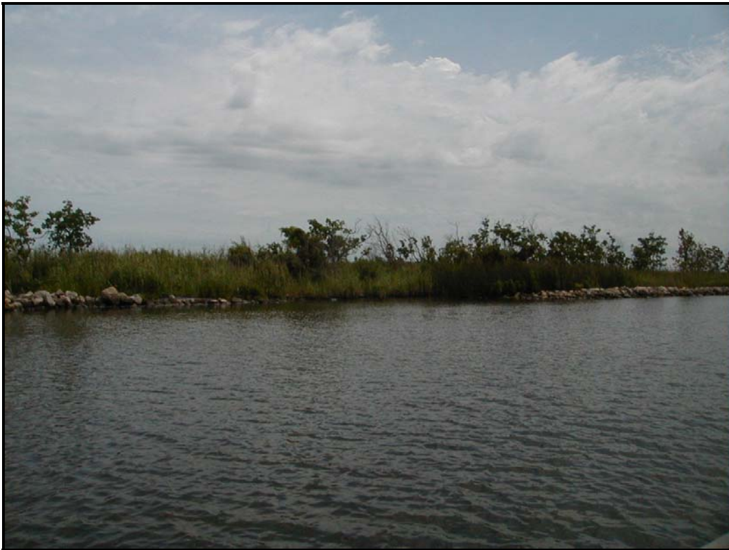
Photo 2, Rock dike, view showing low area hit by barge.
