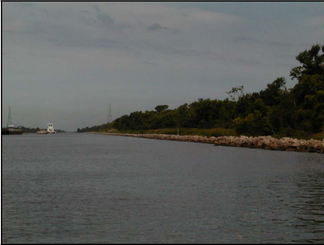
Photo 1, Typical rock dike.
