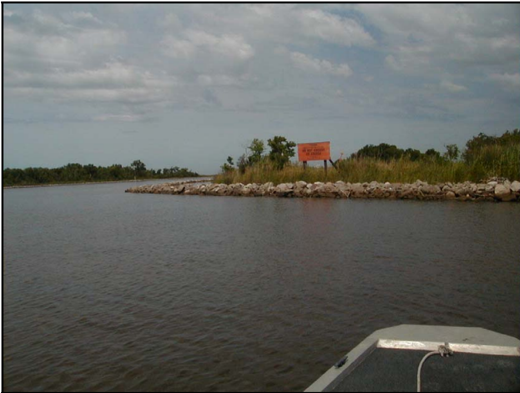
Photo 2, Rock dike tie-in.
