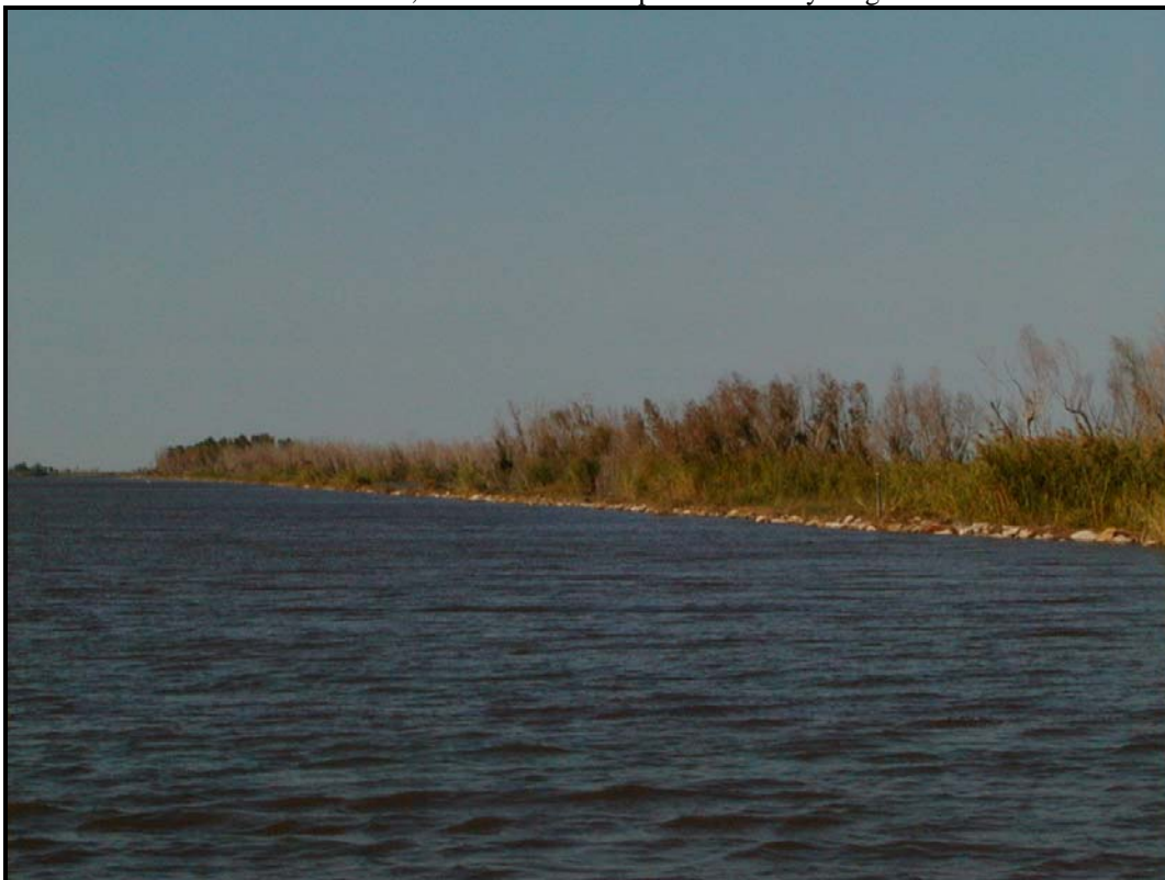
Photo No.2, Typical rock dike section.
