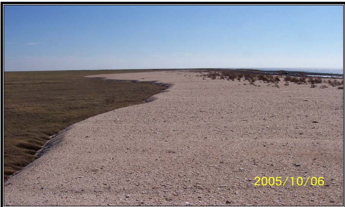
TE-22 – photo of accumulation of sand material behind the rock dike along the Gulf of Mexico adjacent to the rock plug at the end of Transco Pipeline Canal.
