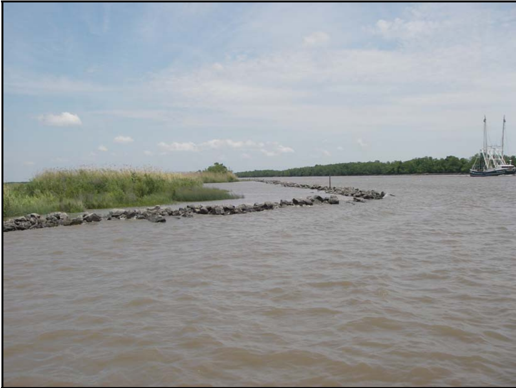
Photo 2, rock dike southern tie-in
