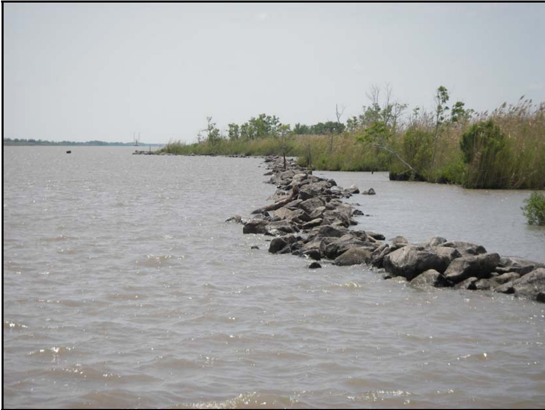
Photo 1, rock dike northern tie-in
