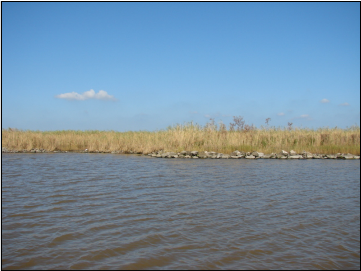
Photo No. 1, Typical rock dike
