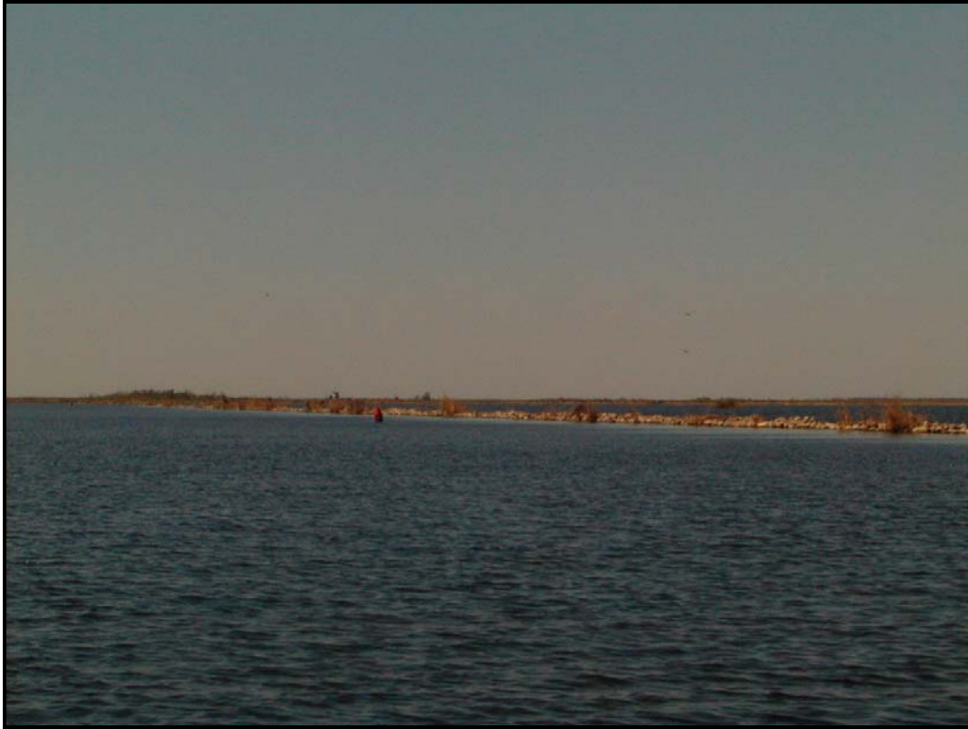
Photo No. 1, Typical rock dike
