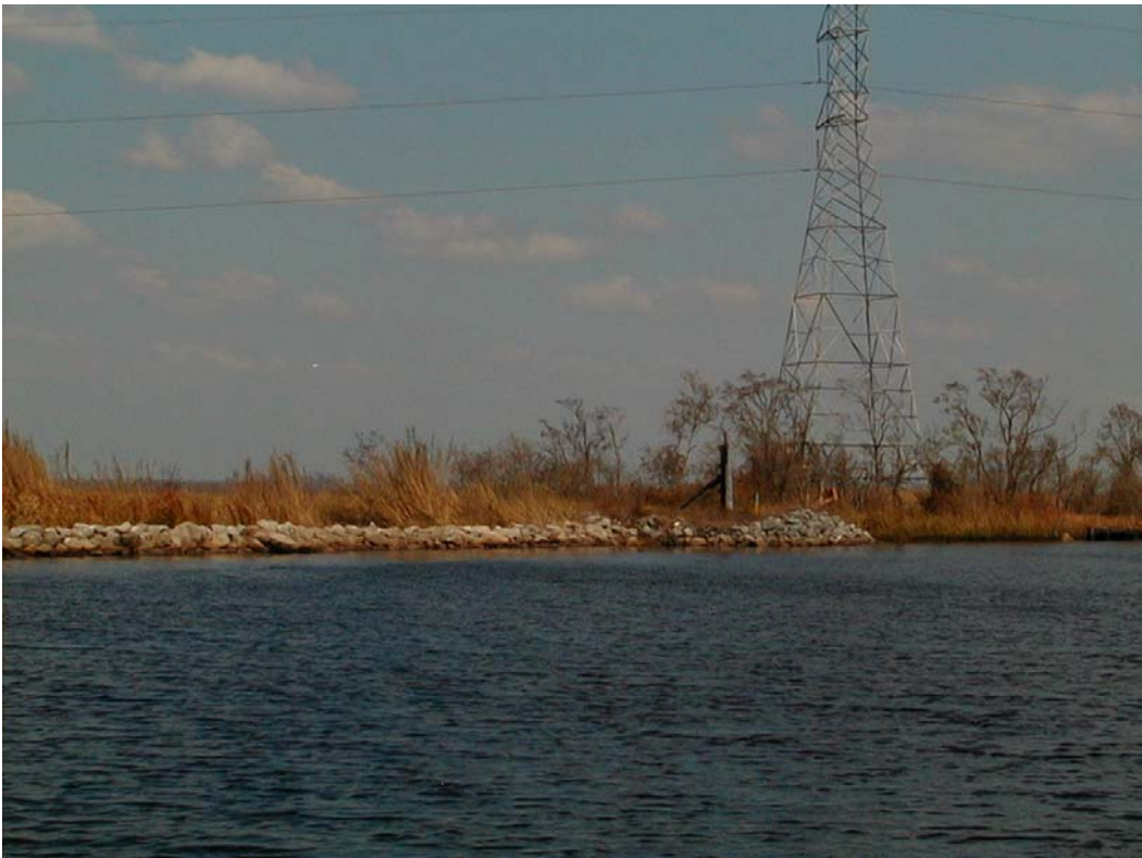
Photo 2, Rock dike tie-in.
