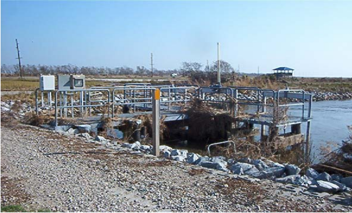
Photo 3, Headquarters' Canal Structure
