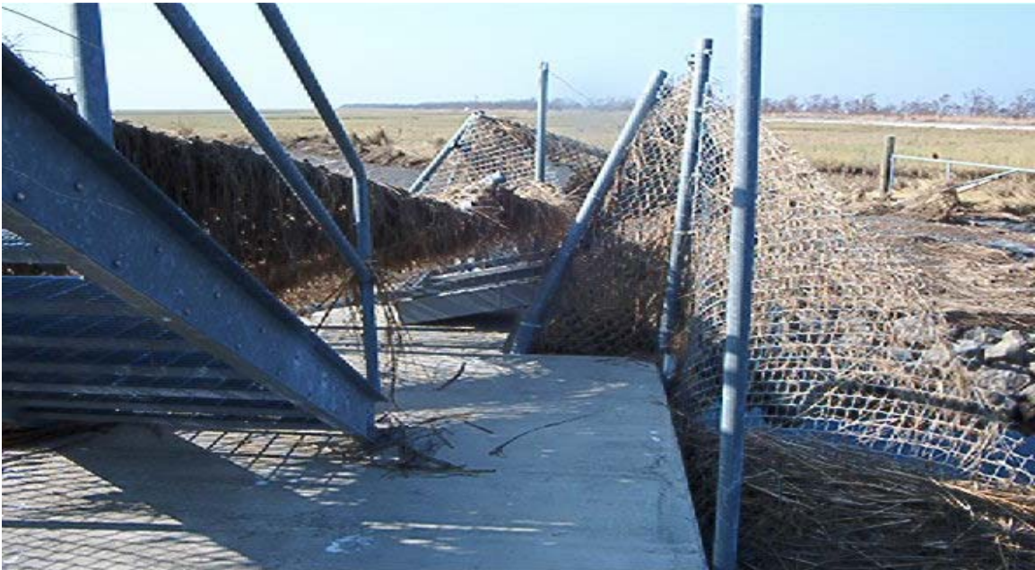
Photo 2, South Walkway On Hog Island Gully Structure
