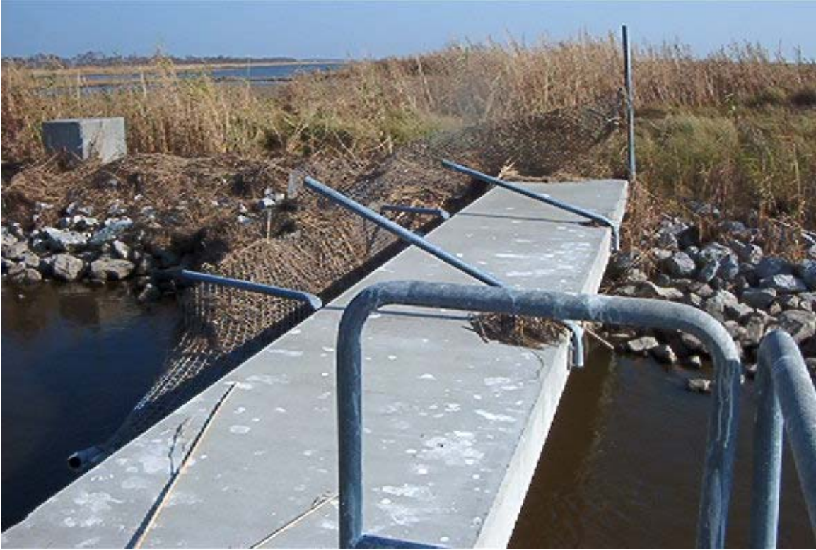
Photo 1, North Walkway On Hog Island Gully Structure
