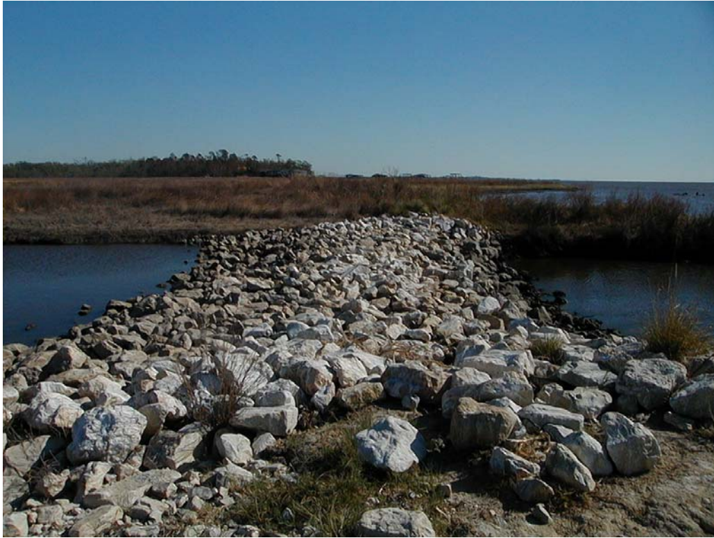
Photo 7, Rock plug at structure No. 8, view looking south.
