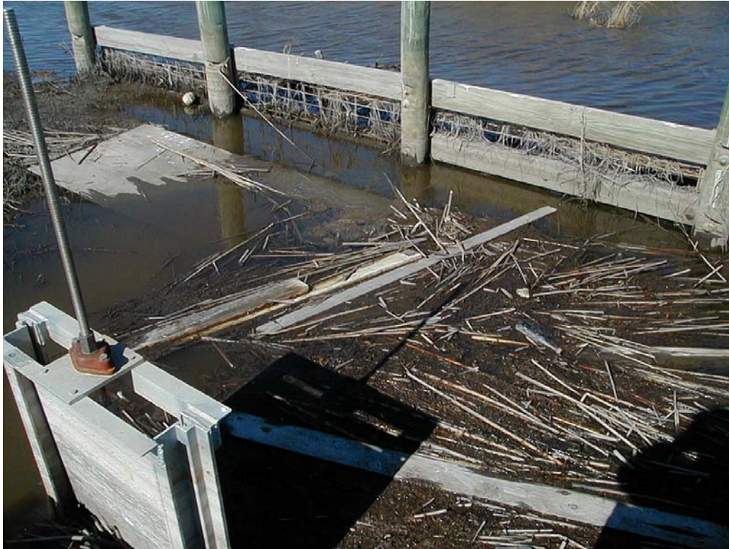
Photo 1, View showing hyacinth fence and sluice gate at structure No.1
