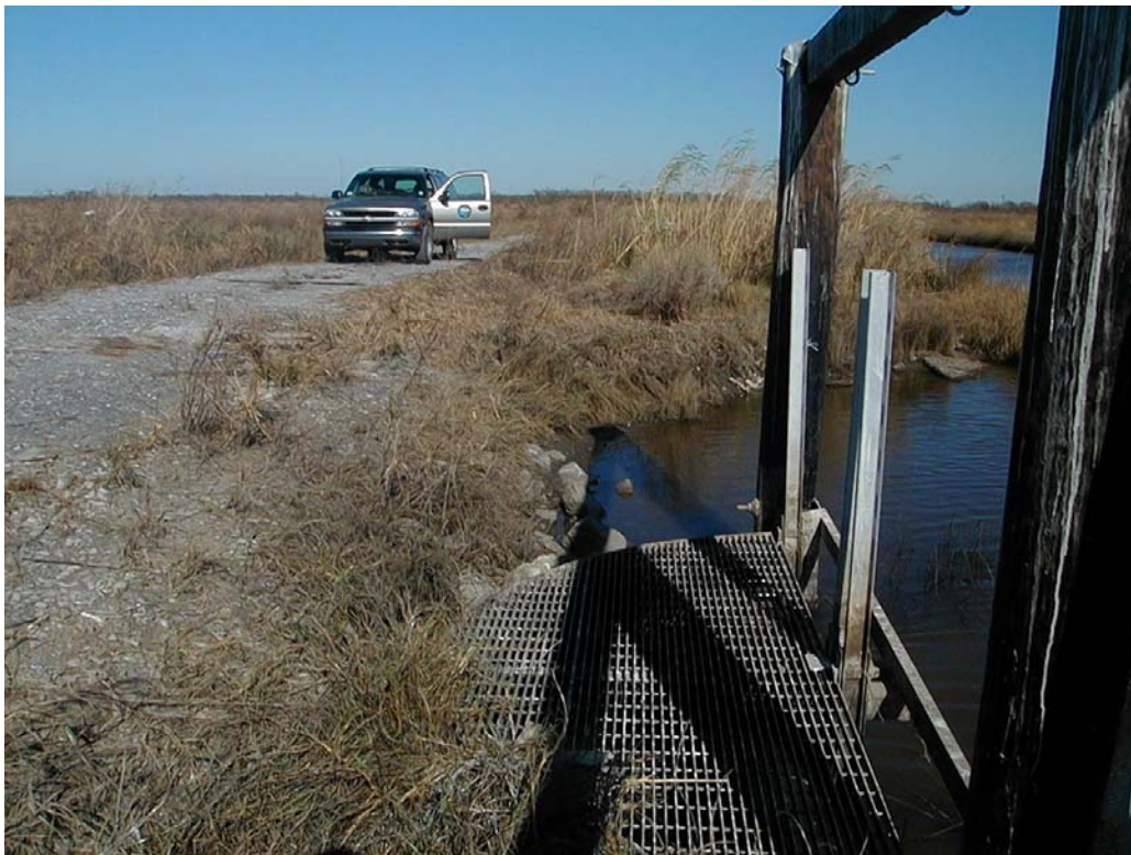
Photo 4, Inlet side of structure No. 12.
