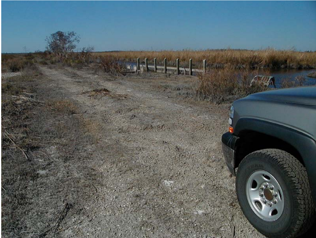
Photo 3, View of roadway approaching structure No. 1.
