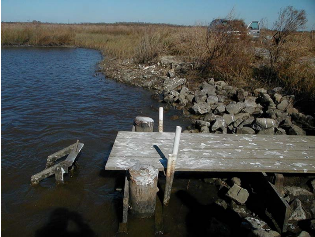
Photo 5, Outlet side of structure No. 12.
