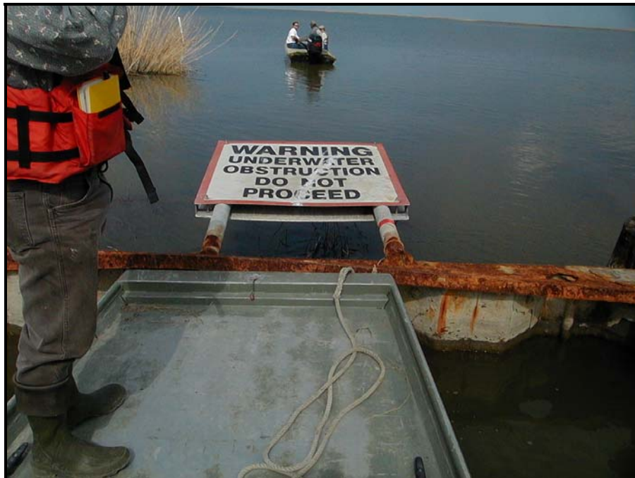
Photo 14, Structure No. 17, showing bent warning sign and damaged pile cap.
