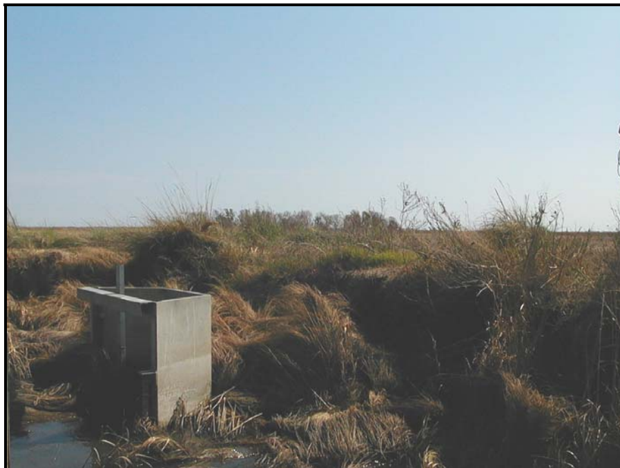
Photo 12, Structure No. 3, showing marsh debris/siltation in and around the structure.
