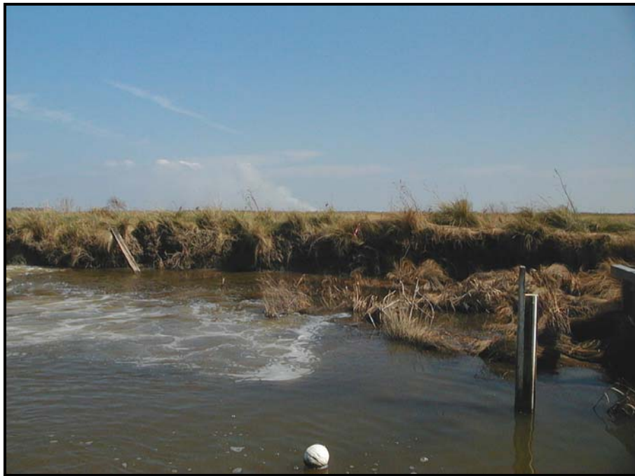
Photo 11, Structure No. 3, November – 2005, showing additional erosion along structure and eastern levee.
