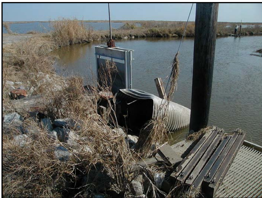
Photo 4, Structure 9a & 9b, showing metal culvert debris lodged on structures.
