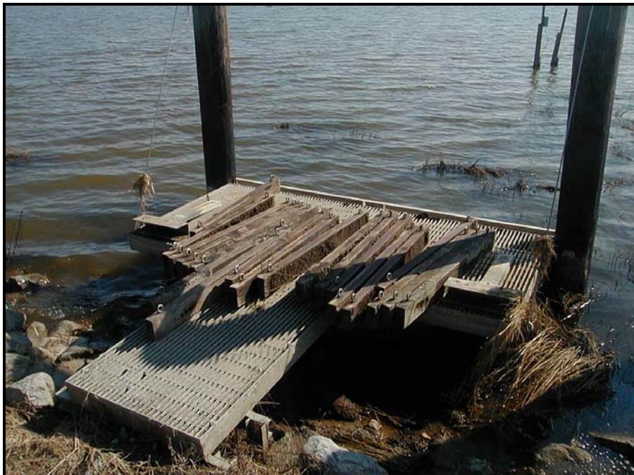
Photo 2, Structure No.7 showing marsh debris/siltation and minor erosion at grate.
