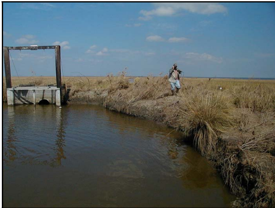
Photo 8, Structure No. 5, November -2005, showing additional bankline erosion along structure and on eastern levee.
