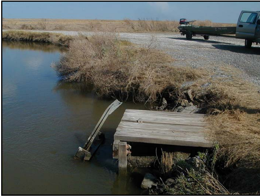
Photo 5, Structure 9b, showing broken flapgate handle.
