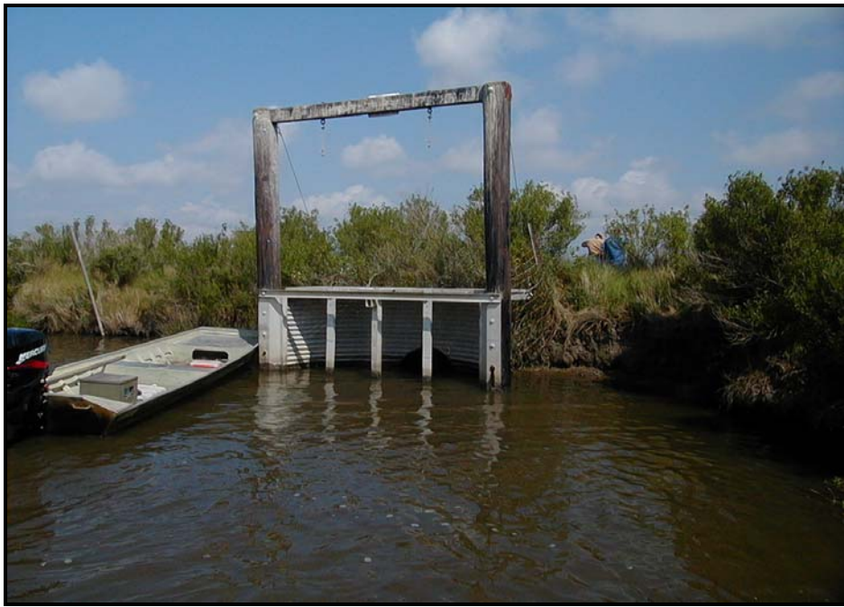
Photo 7, Structure No. 5, March – 2005, showing bankline erosion.
