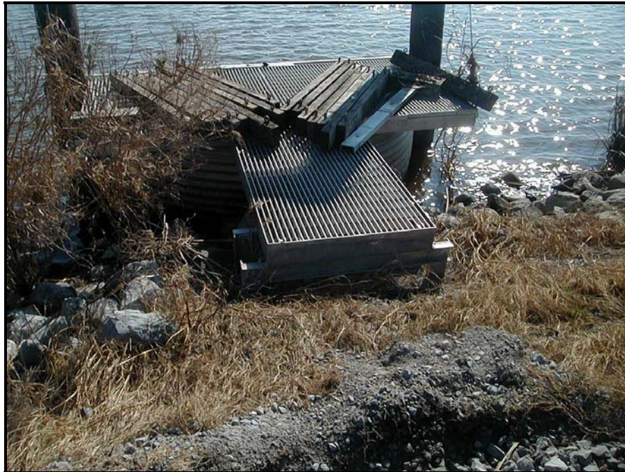
Photo 1, Structure No. 6 showing erosion at end of grating.
