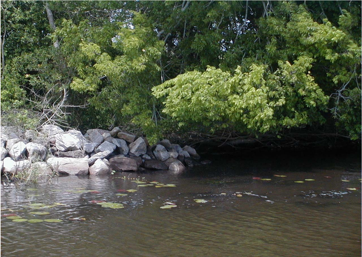
Photo 1—southern tie-in on Burton Sutton Canal (April 21, 2005)
