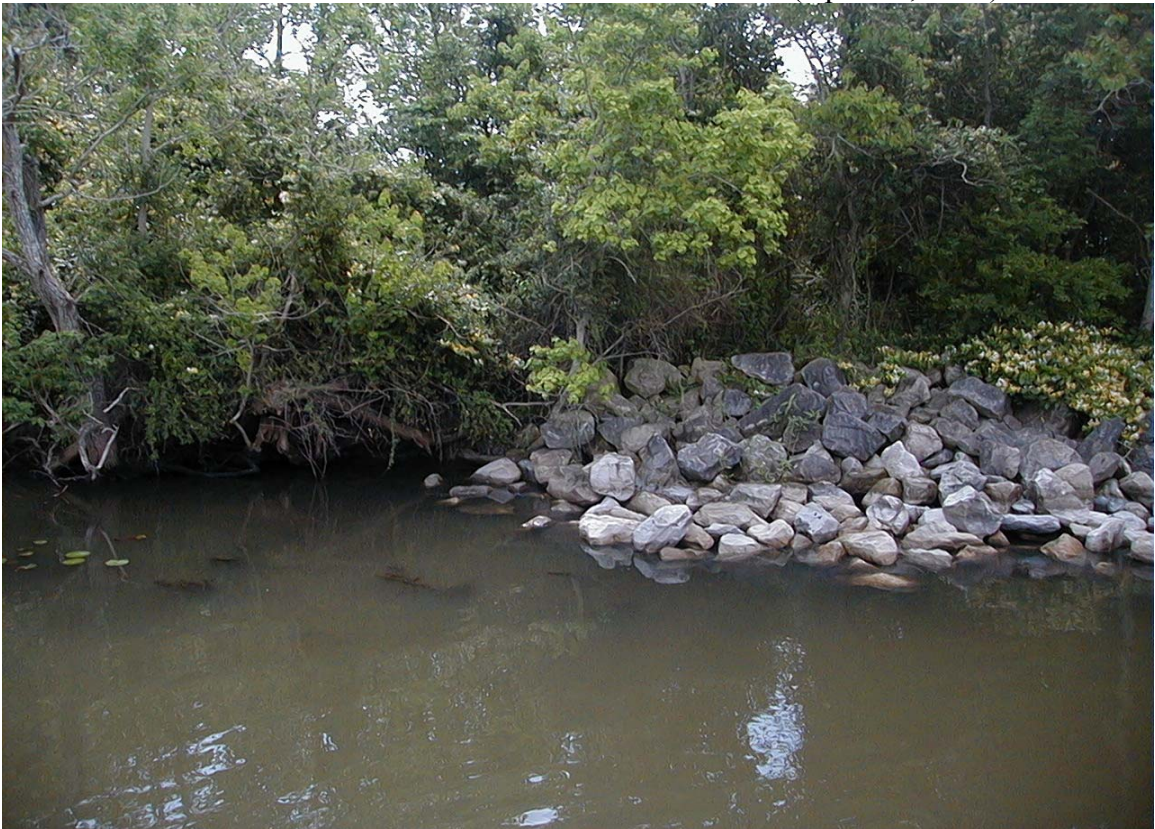
Photo 2—northern tie-in (April 21, 2005)
