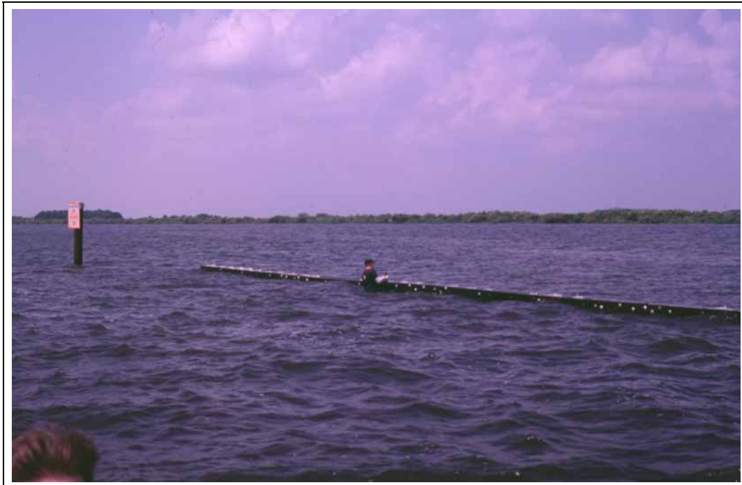
Figure 9. Typical Vinyl Sheet Pile structures at the Lake Salvador Shoreline Protection (BA-15) Demonstration project (photo taken in December 1998).
