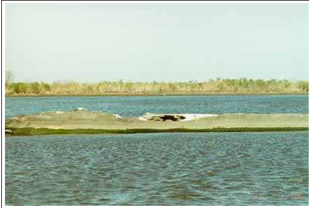
Figure 20. Typical damage exhibited by the Geotextile tube structures at the Lake Salvador Shoreline Protection (BA-15) Demonstration project (photo January 2000).
