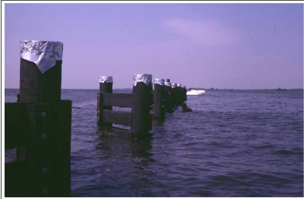
Figure 8. Typical Angled Timber Fence structure at the Lake Salvador Shoreline Protection (BA-15) Demonstration Project (photo taken December 1998).
