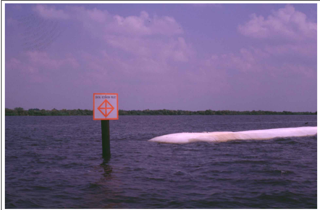
Figure 7. Typical geotextile tube structure at the Lake Salvador Shoreline Protection (BA-15) Demonstration project (photo taken December 1998).
