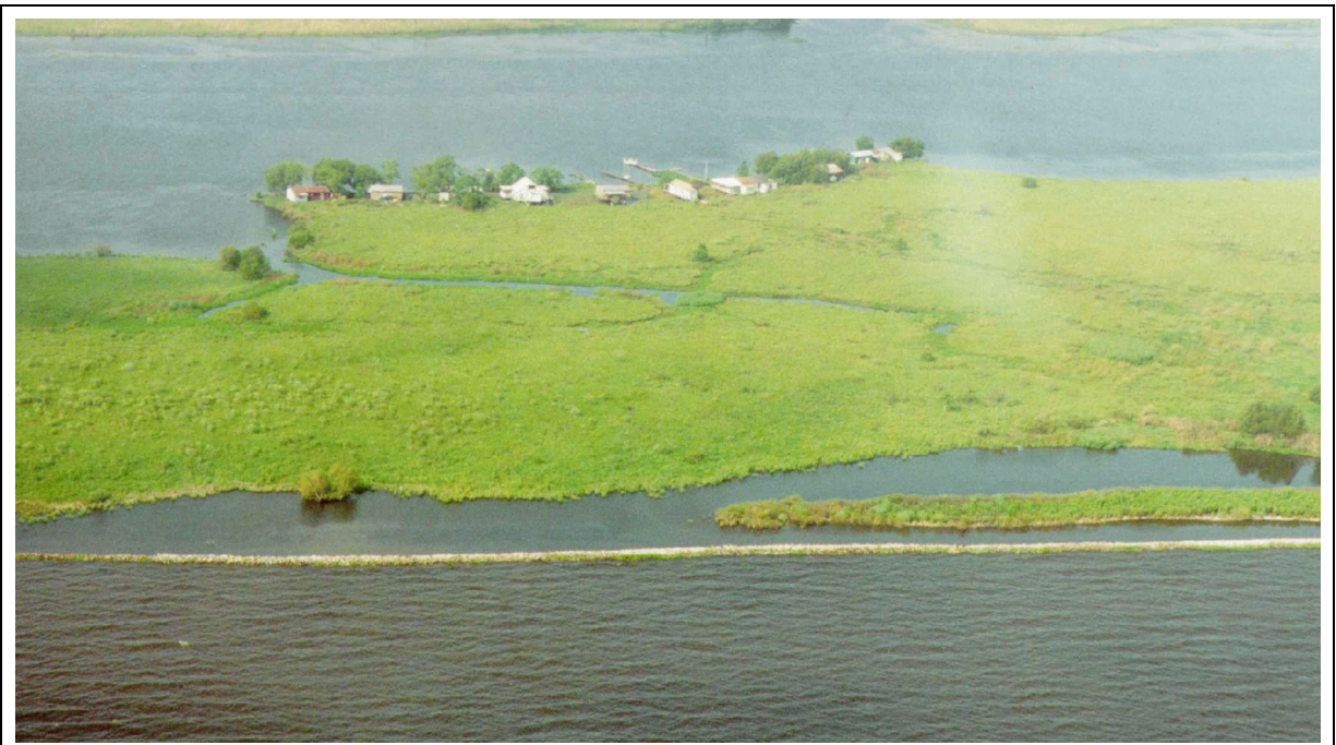
Figure 10. Typical rock berm structure at Lake Salvador Shoreline Protection (BA-15) Demonstration project (photo taken August 1998).
