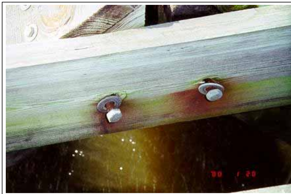
Figure 23. Typical structural damage exhibited by the Grated Apex and Angled Timber Fence structures at the Lake Salvador Shoreline Protection (BA-15) Demonstration project (photo January 2000).
