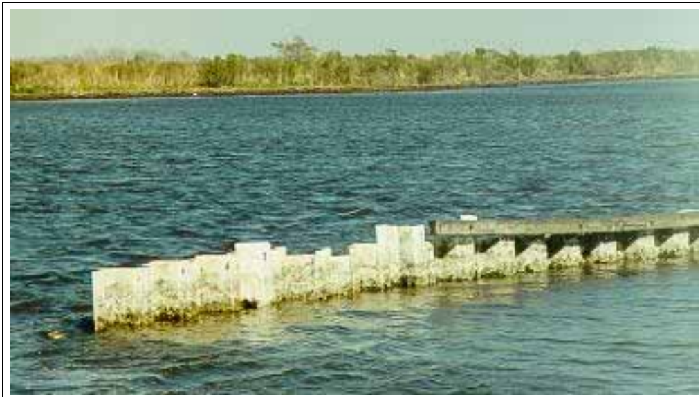
Figure 21. Typical structural damage to the unreinforced Vinyl Sheet Pile structures at the Lake Salvador Shoreline Protection (BA-15) Demonstration project (photo January 2000).
