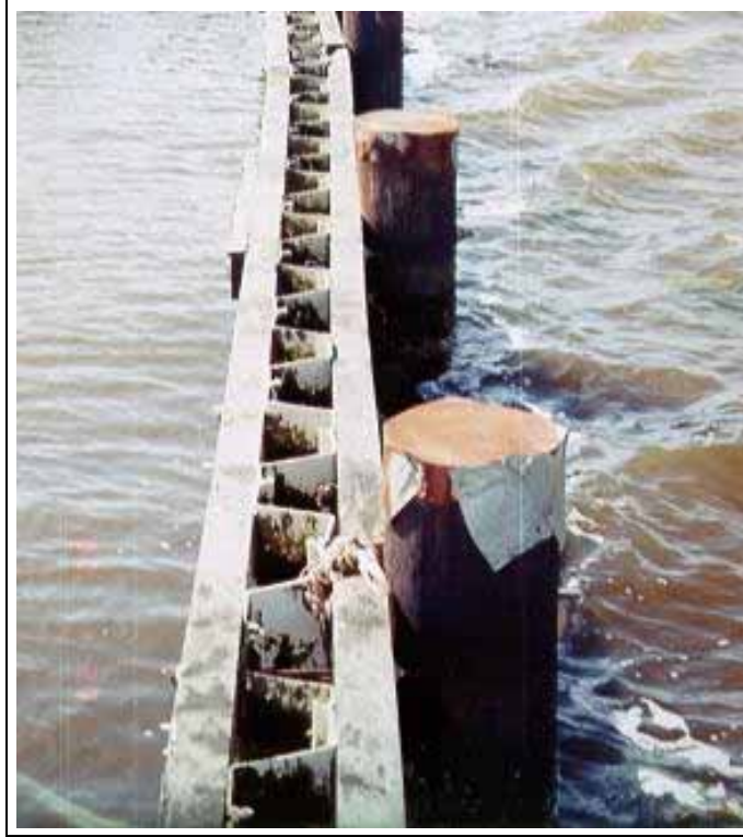
Figure 22. Typical structural stability of the reinforced Vinyl Sheet Pile structure the Lake Salvador Shoreline Protection (BA-15) Demonstration project (photo January 2000).
