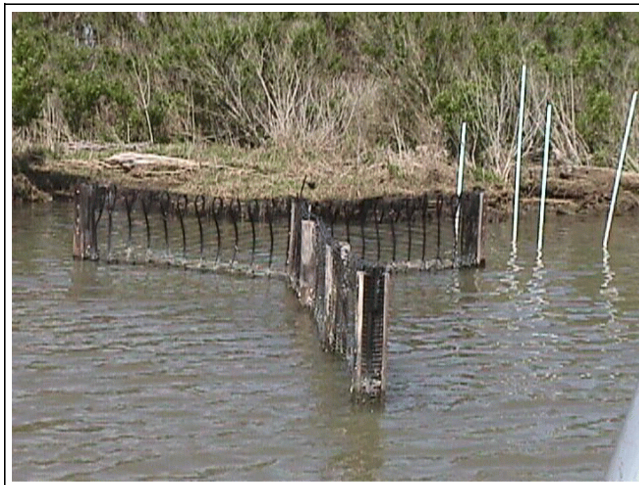
Figure 7. Shore-perpendicular, five and four section uniaxial geo-gid fence with flared end (design C) at Falgout Canal - Vegetative Plantings Demonstration Project (TE-17) (Photo taken March 13, 2000).
