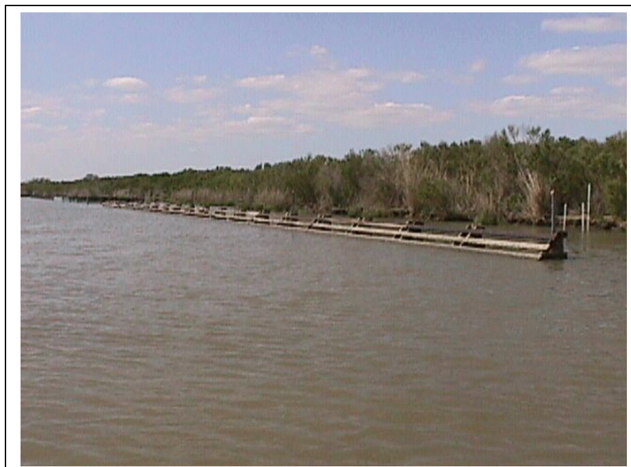
Figure 6. Shore-parallel single sided wooded A-frame (design B; treatment 7) at Falgout Canal - Vegetative Plantings Demonstration Project (TE-17) (Photo taken March 13, 2000).
