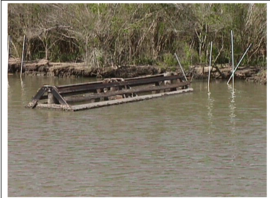
Figure 5. Shore perpendicular, four and five section double sided wooden A-frame (design A; treatments 1 and 8) at Falgout Canal - Vegetative Plantings Demonstration Project (TE-17) (Photo taken March 13, 2000).
