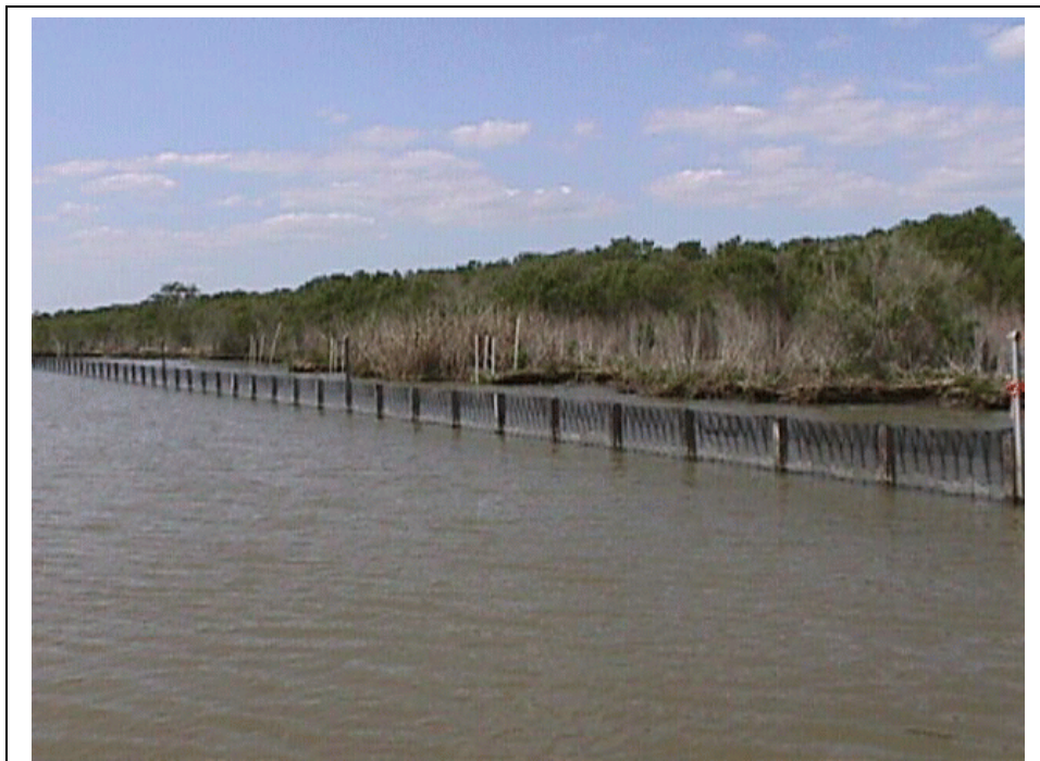
Figure 9. Shore-parallel, uniaxial geo-grid fence (design E; treatment 5) at Falgout Canal - Vegetative Plantings Demonstration Project (TE-17) (Photo taken March 13, 2000).
