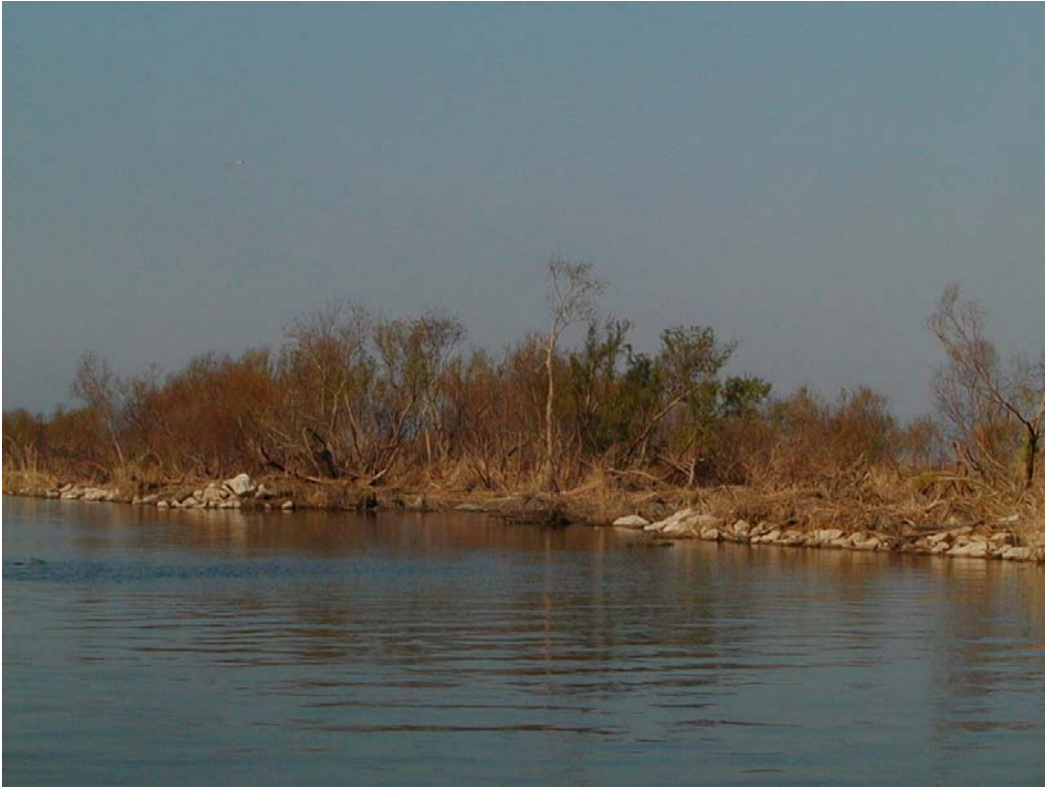
Photo No.1, Area of rock dike pushed back by barge.
