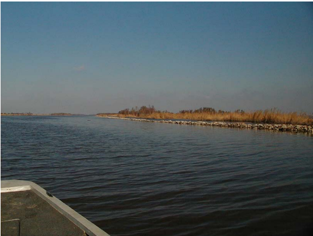
Photo No.2, Typical rock dike section.
