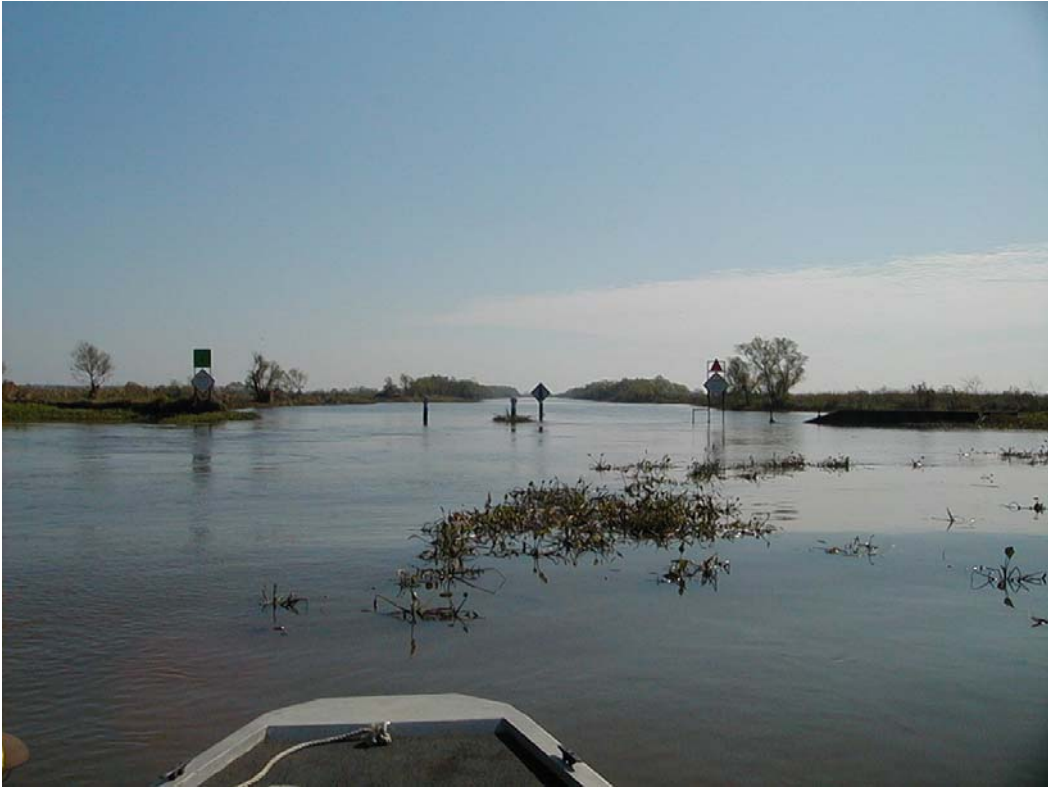
Photo 1, Mud Bayou Structure
