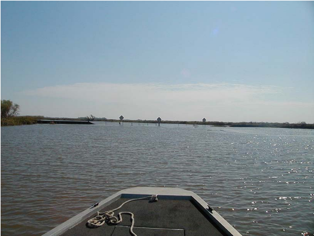
Photo 2, Humble F-Canal Structure
