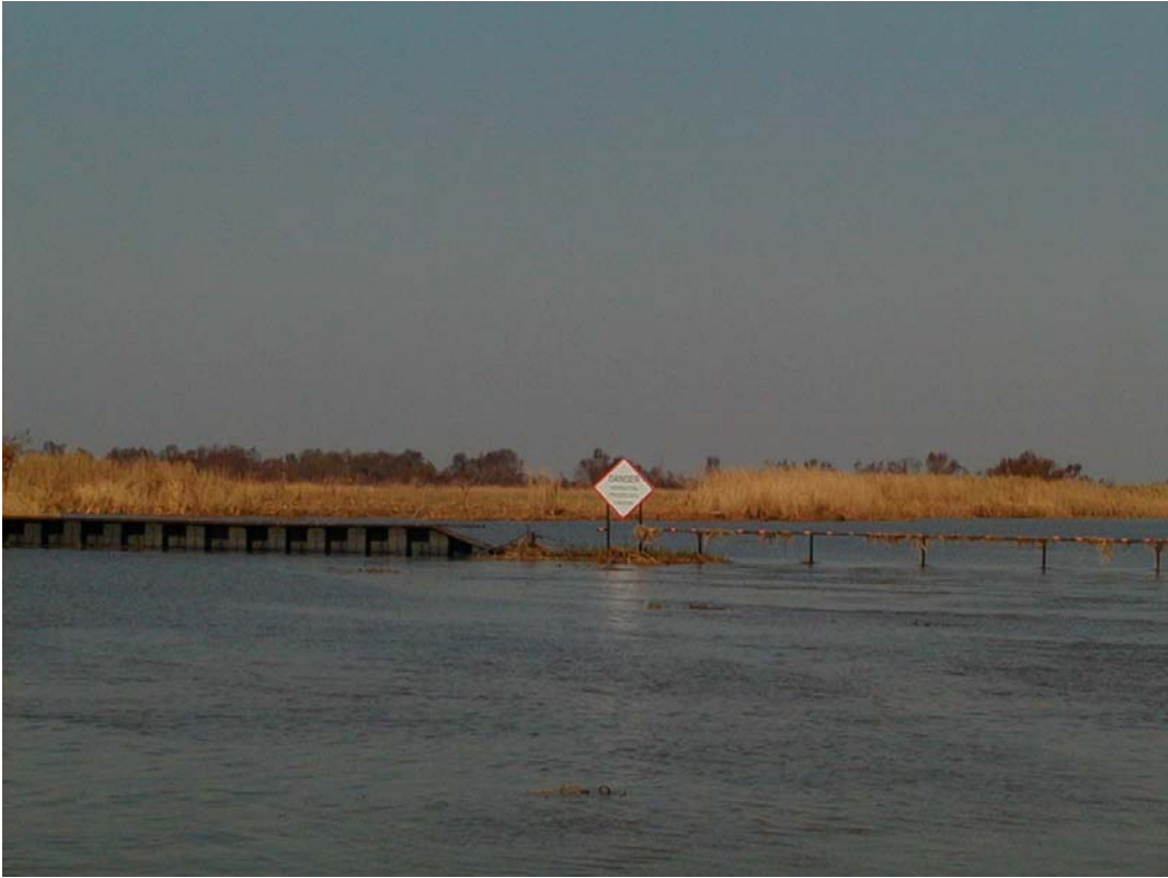
Photo 5, Humble Canal Structure
