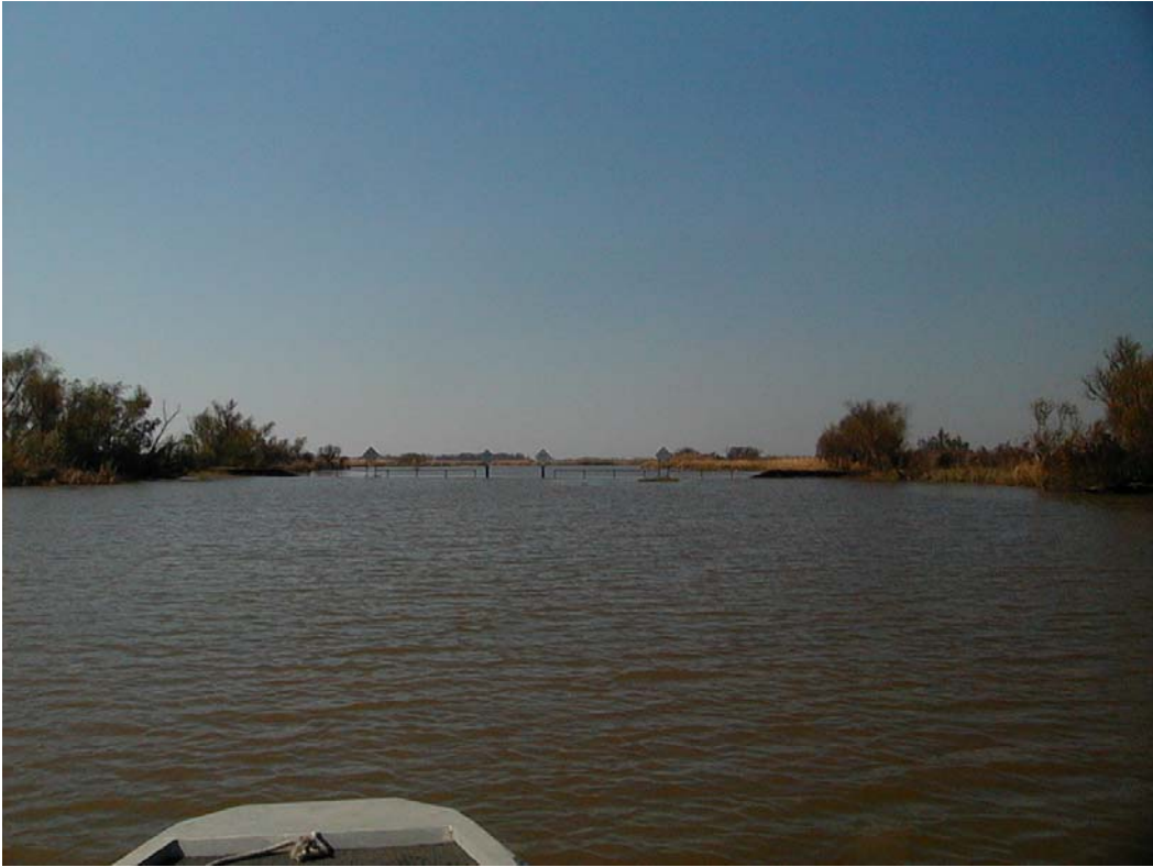
Photo 3, Bayou Long Structure
