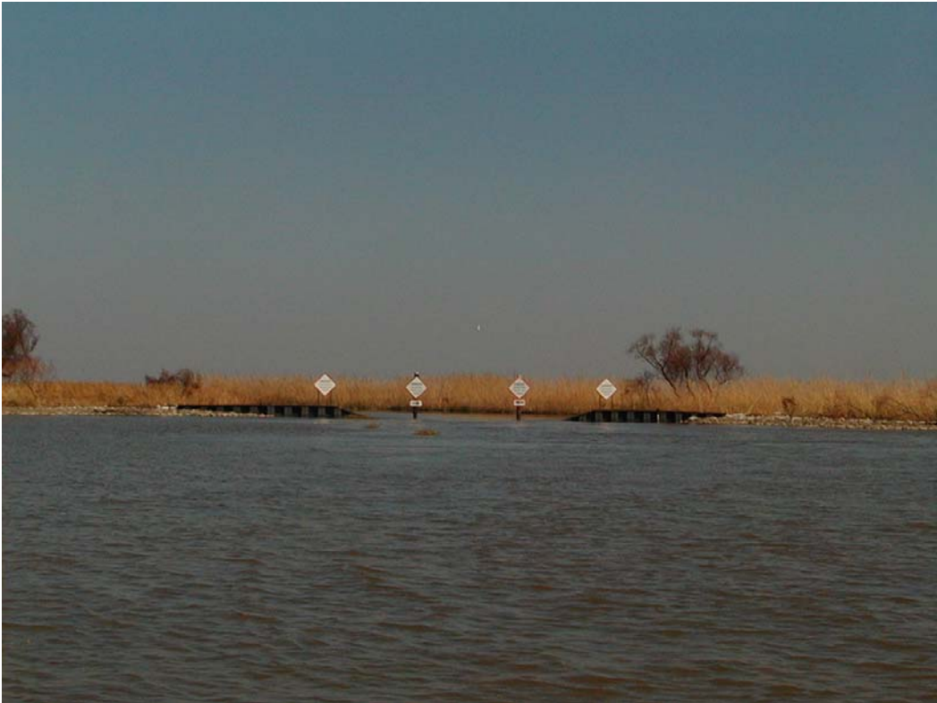
Photo 8, Jackson Bayou Structure
