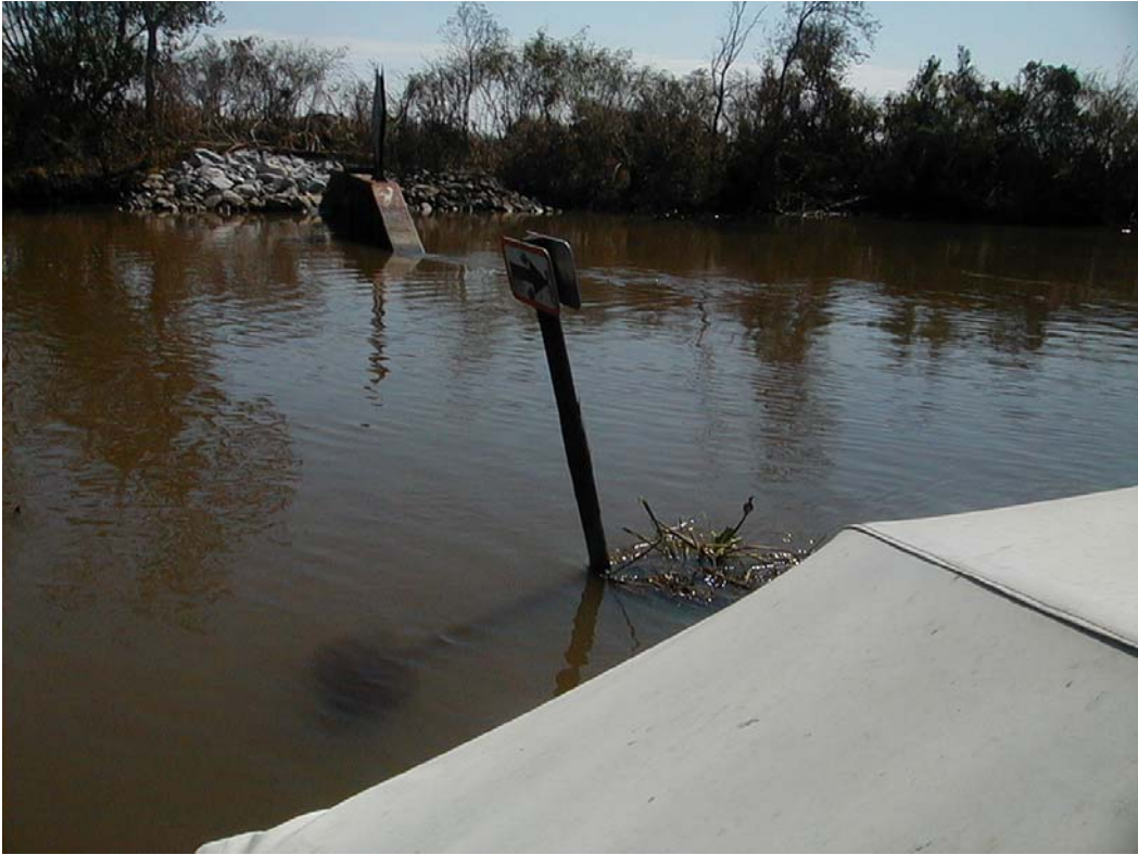
Photo 11, British American Canal Structure
