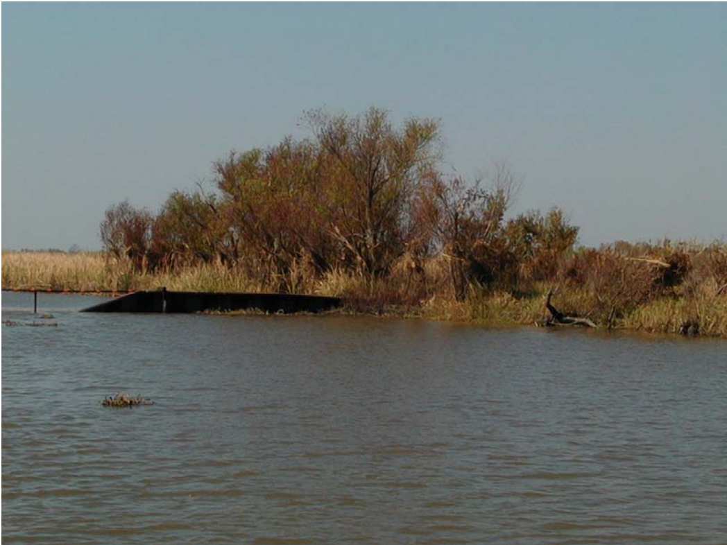
Photo 4, Bayou Carlin Structure
