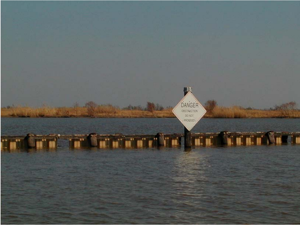
Photo 9, PVC Sheet Pile Wall
