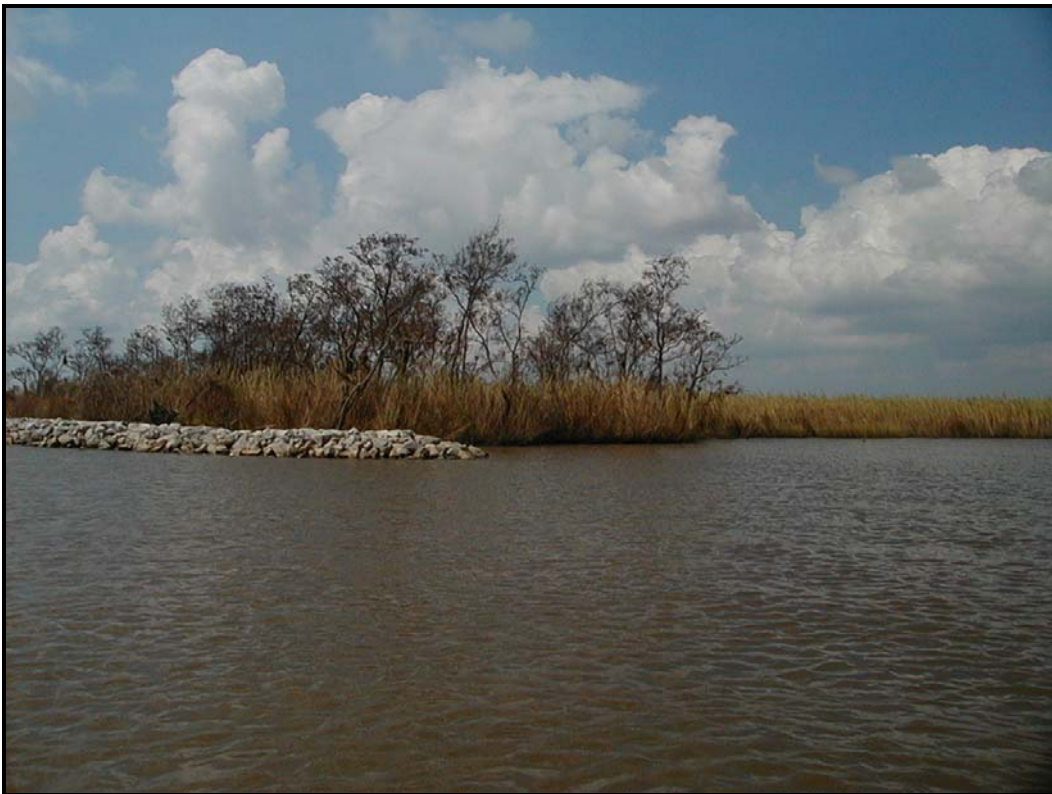
Photo 2, Rock tie-in on southern end of project.
