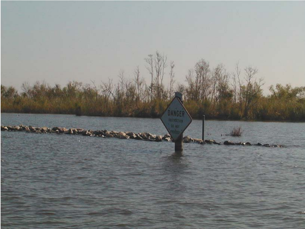
Photo 1, Typical rock dike, note high water from Hurricane RITA storm surge.
