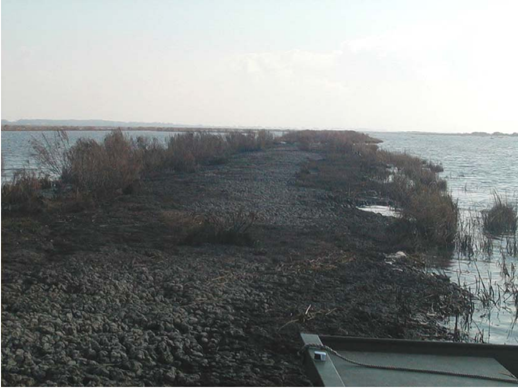
Photo 1, Typical earthen terrace.
