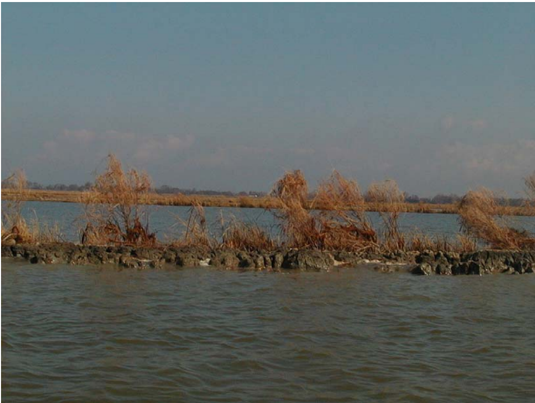
Photo 2, Typical eroded terrace.
