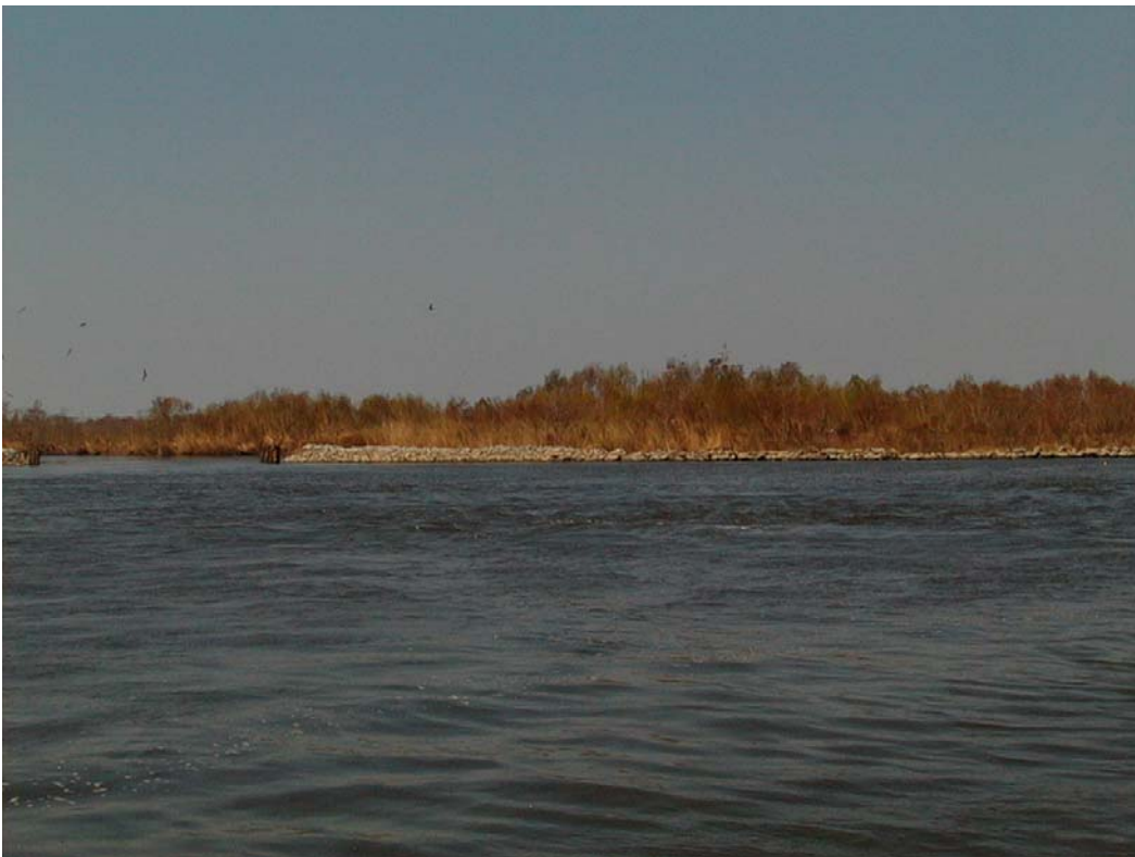
Photo 2, Typical rock dike.
