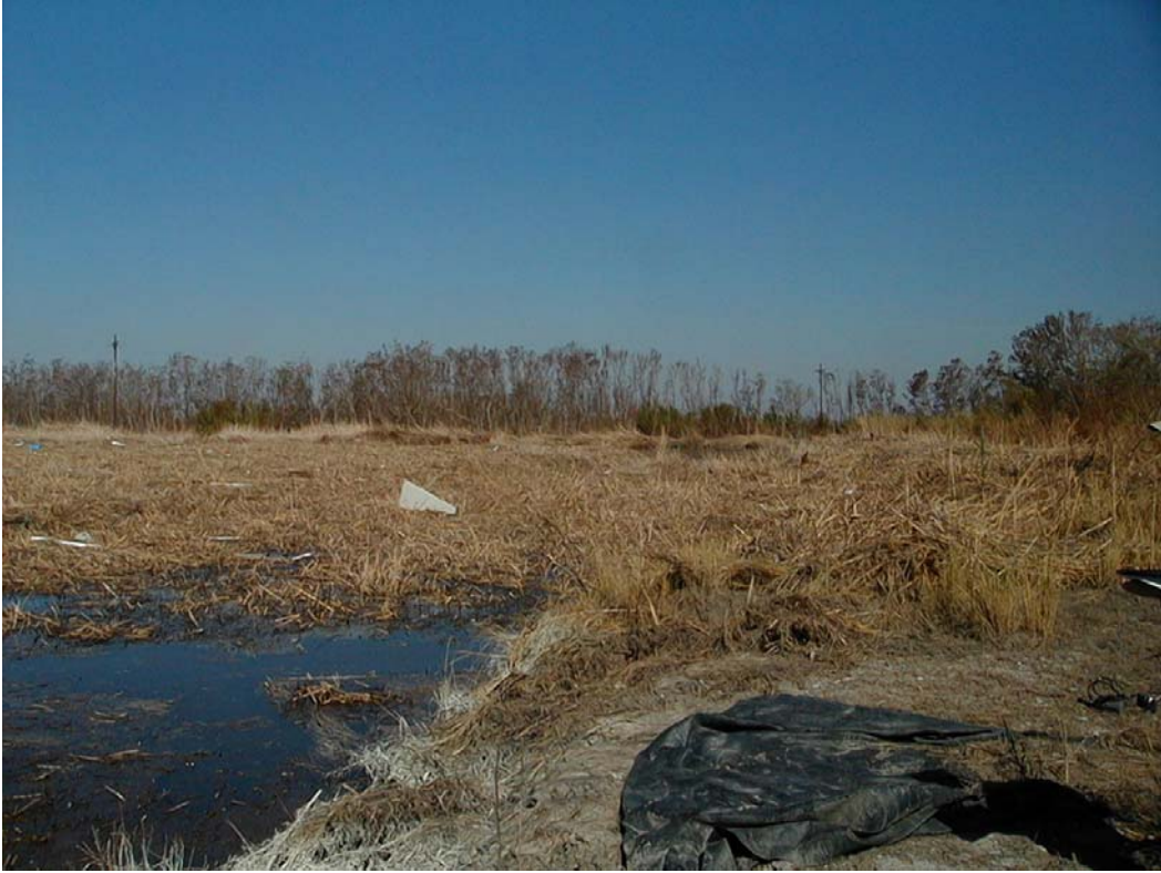
Photo 5, Showing clogged inlet channel, view looking north.
