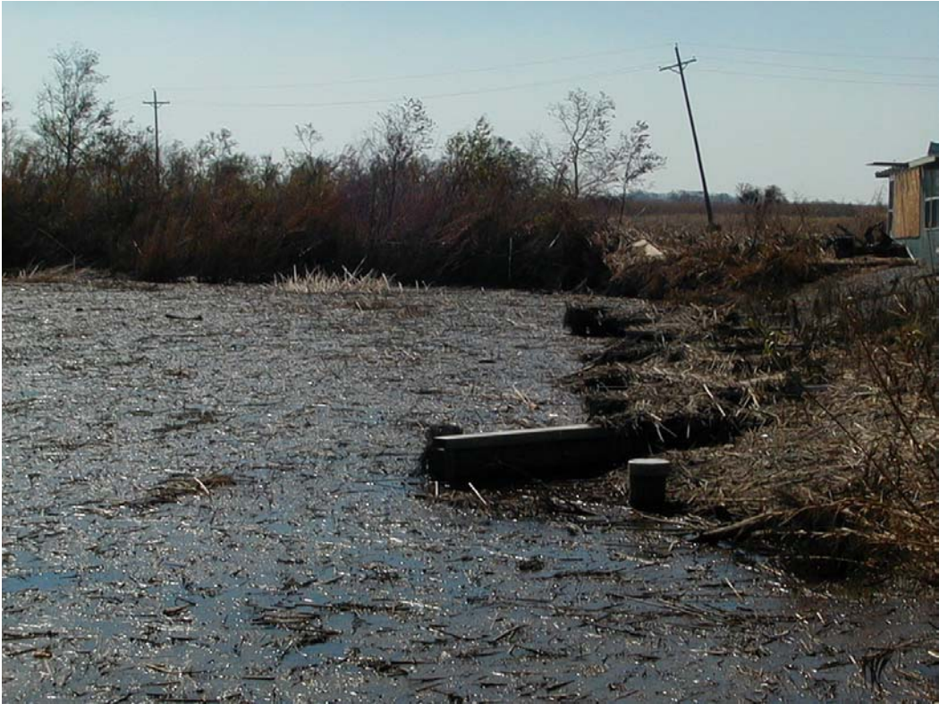
Photo 3, Outlet side of structure covered with wrack.
