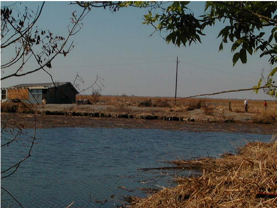
Photo 4, Showing camp on southern end of structure embankment.
