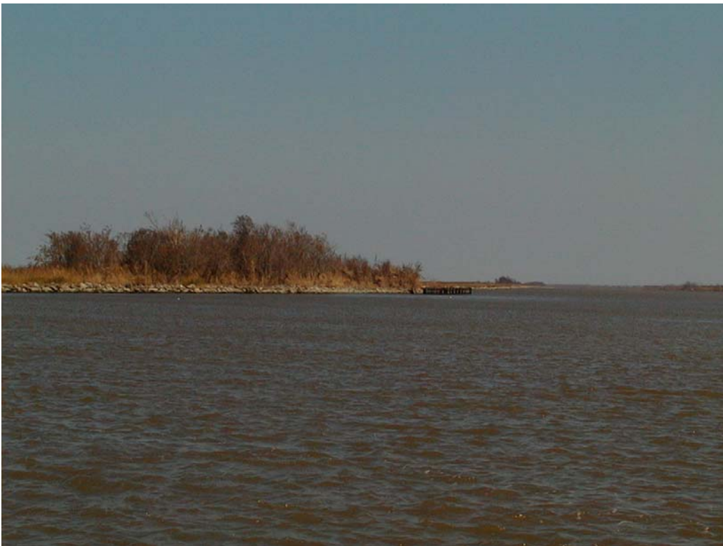
Photo 2, Typical rock dike.
