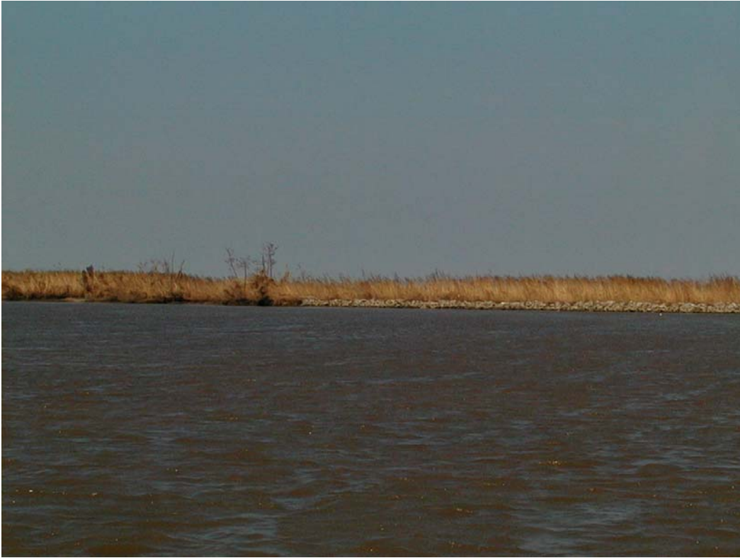
Photo 1, Typical rock dike
