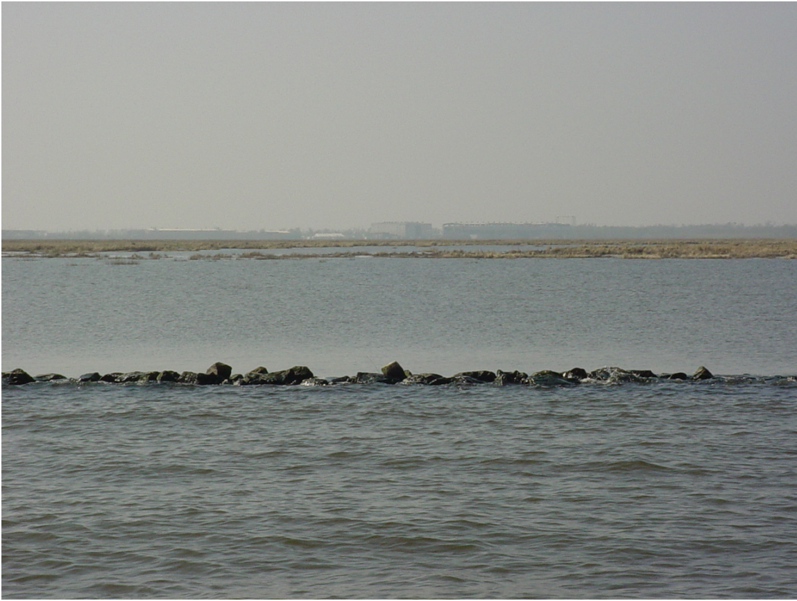
Photo #1 – Rock Dike. Looking toward the project area from Lake Pontchartrain. Notice the difference in surface water activity inside and outside the project area.
