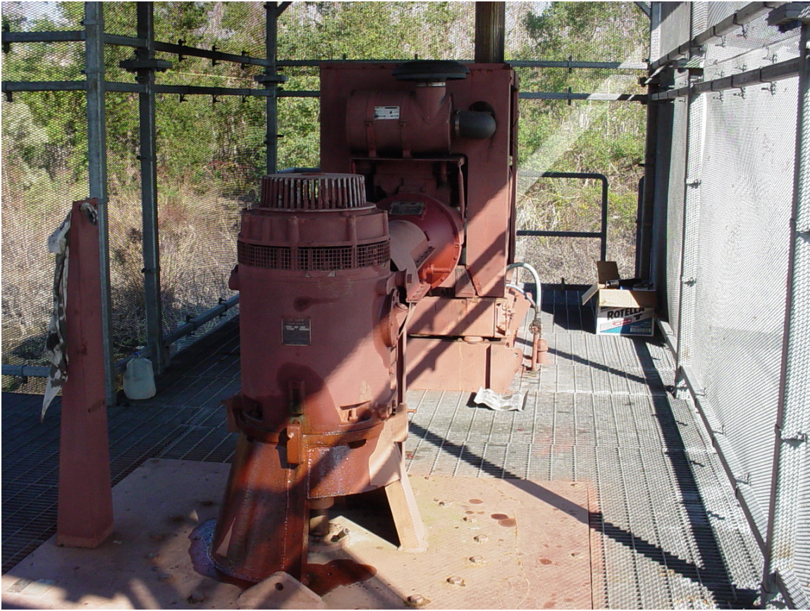
Photo #1 – Pump #3. This pump was working until the clutch froze. Note the leaking fluid.
