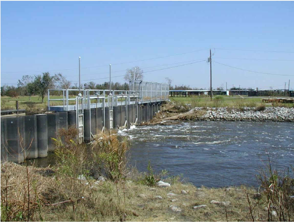
Photo #1 – Water Control Structure.
