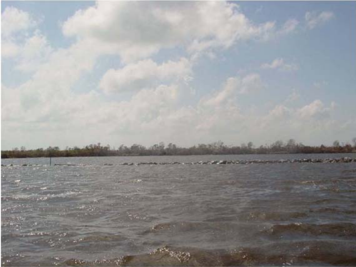
Photo #1 – Shoreline Protection. Before Maintenance Project.
