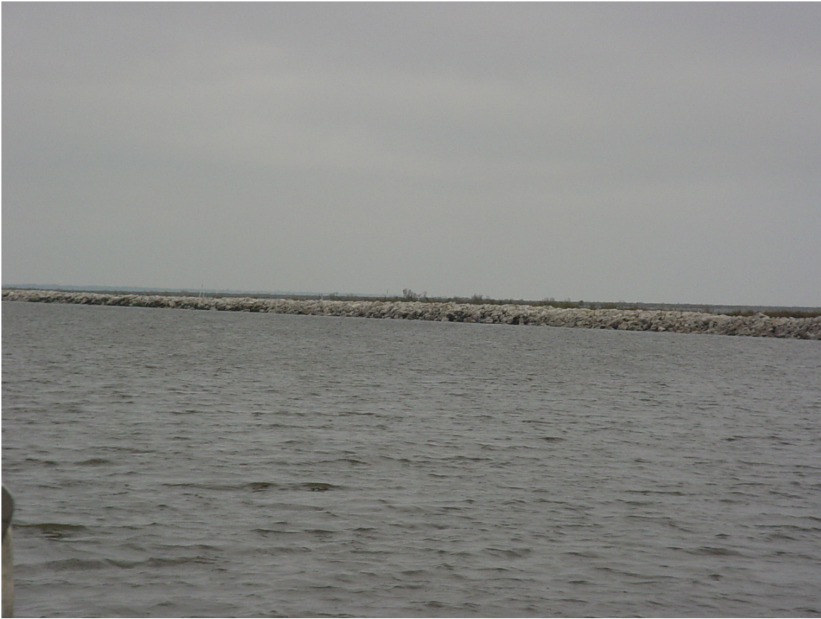
Photo No. 2 – Shoreline Protection. After Maintenance Project.
