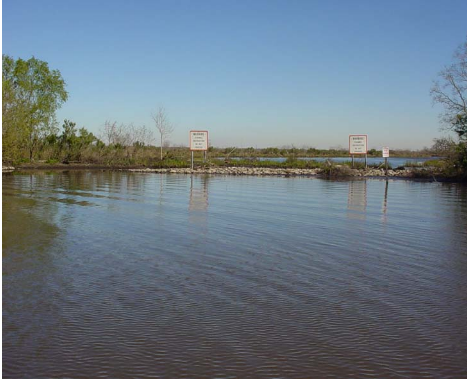
Photo #1 Structure #14, Notice low spot on left of picture.
