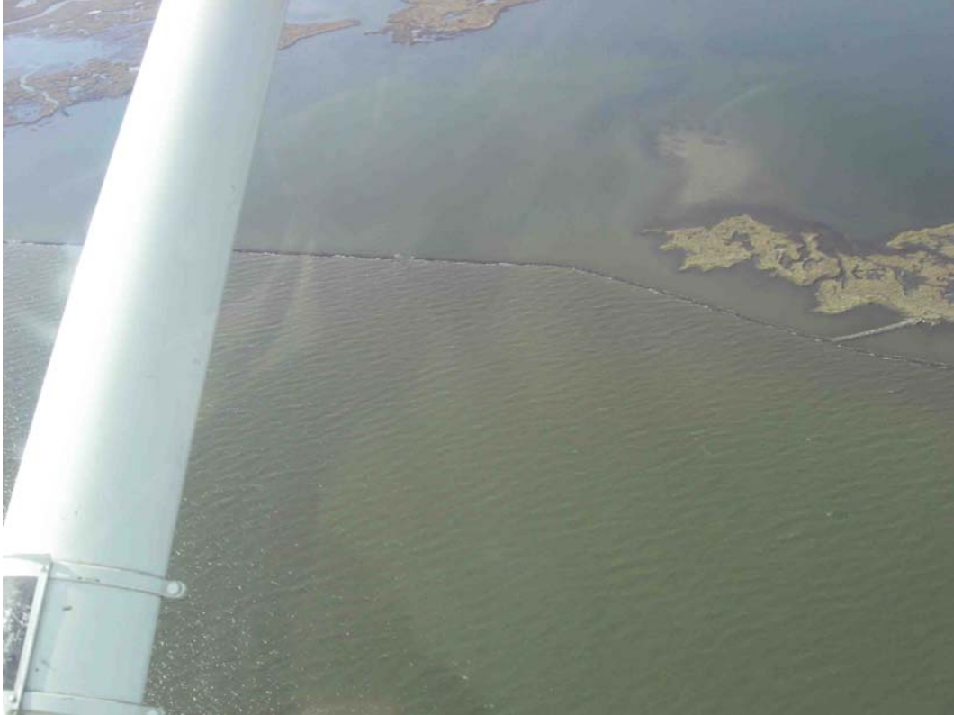
Photo #1 – North Cove Rock Dike.
