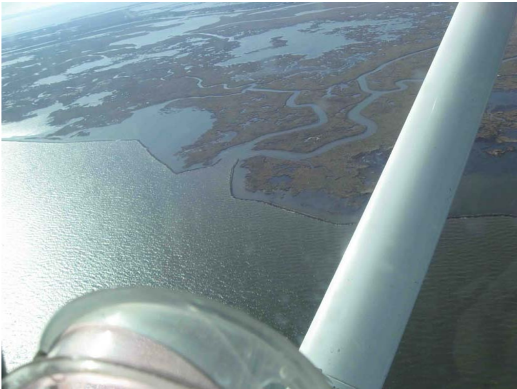
Photo #2 – Bayou Chevee Rock Dike.
