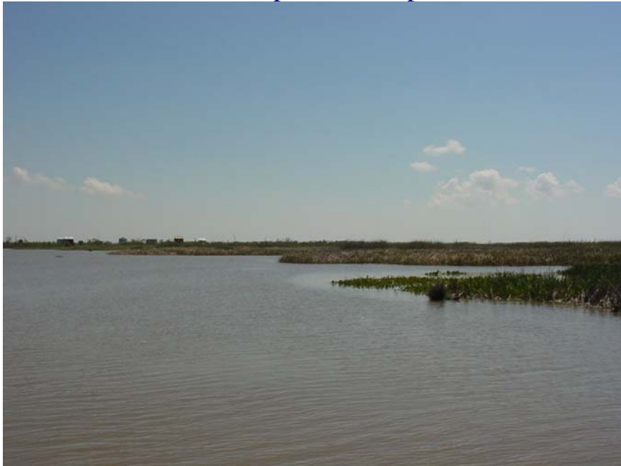
Crevasse No. NC-1, (view 2) Midway into crevasse looking towards vegetated spoil area.
