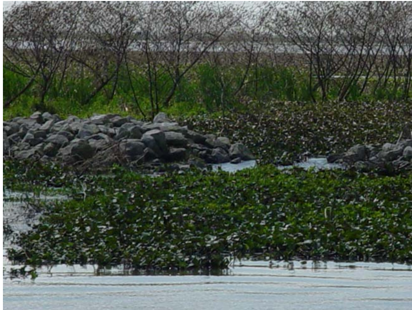
Photo # 6 Site 32 (view 2) Close up view of the vandalized area. Approximately 30% of the west lake rim was destroyed by the storms.
