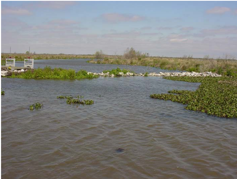
Photo # 19 Site 60(view 1) Slightly more subsidence is noticed in the center part of the rock closure..
