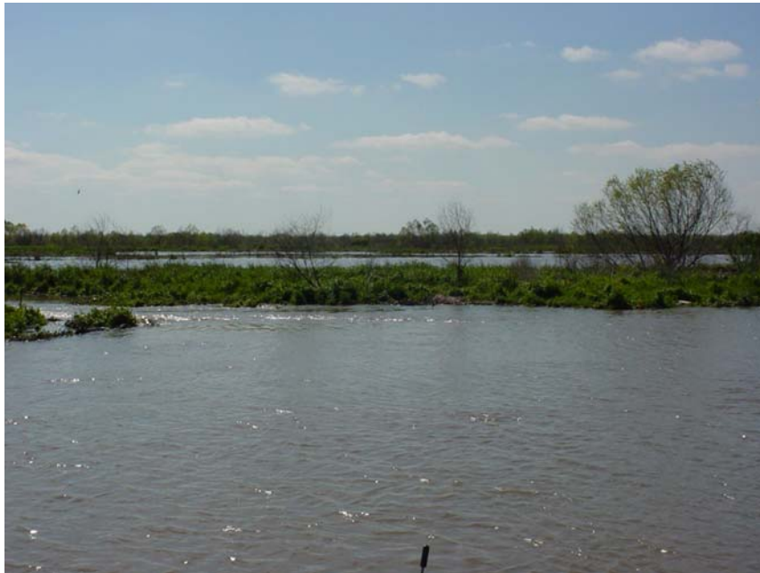
Photo # 10 Site 52 (view 2) This breach in the earthen embankment is approximately 50 yards to the west of the rock plug. Many of these breaches are evident throughout the outfall area allowing free flowage from the conveyance channels into the interior marshes.
