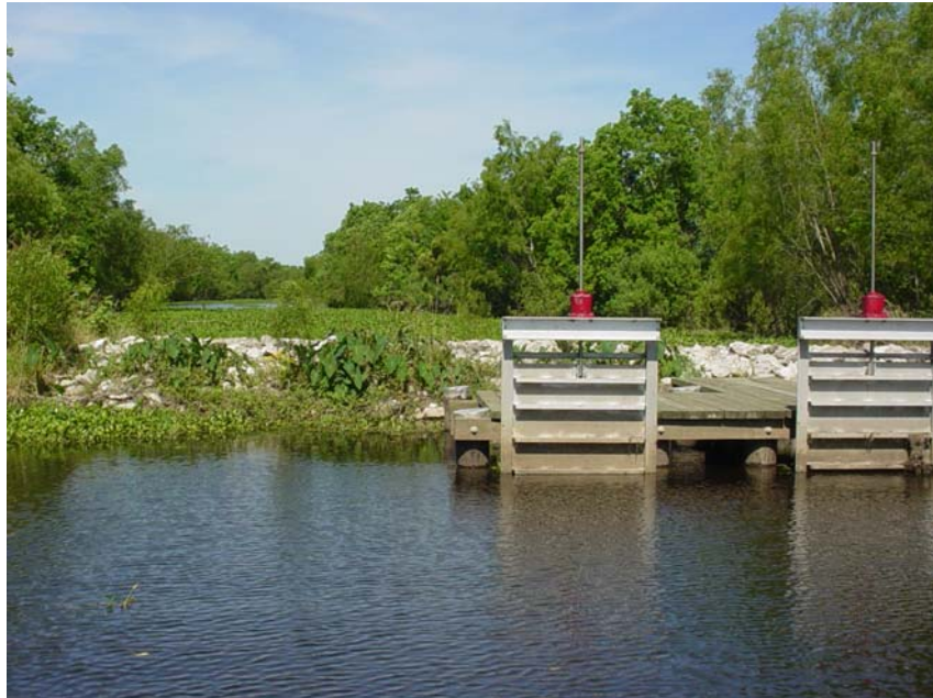
Photo # 3 Site 25 The structure remains covered with storm debris. Both of the gates remained closed to reduce flow to the Braithwaite area where the USACE was constructing an emergency levee contract. That contract has since been completed. This site was not accessible during the 2008 inspection.
