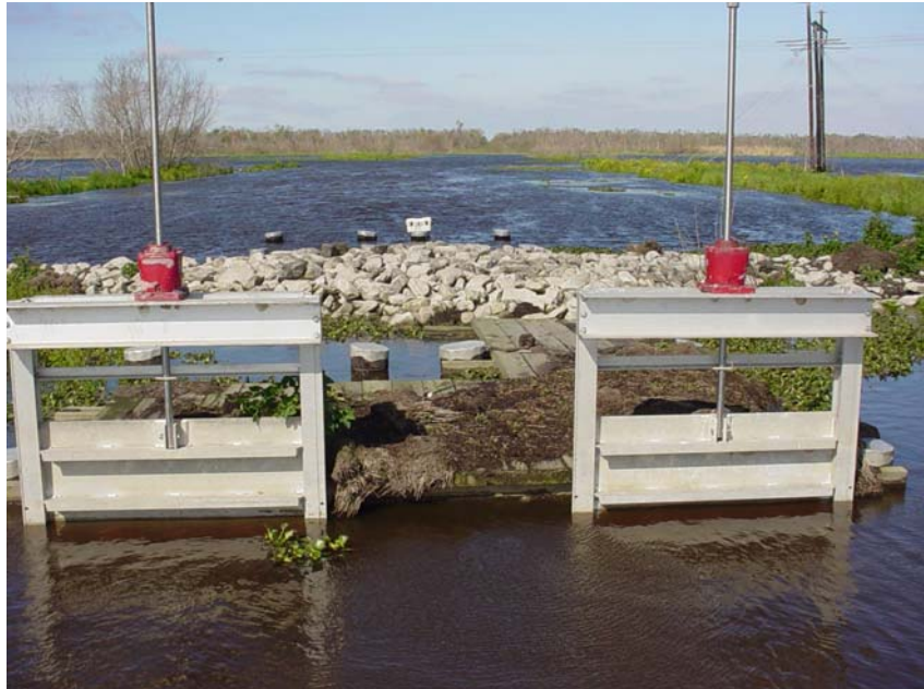
Photo # 7 Site 40 Small amounts of storm debris still remains on structure. The blockage of the culverts by storm debris has been cleared. The flow-meter was damaged but recovered will be replaced. Note the high water stages from the structure westward to the Plaquemines east bank hurricane levee (tree line) in the background.
