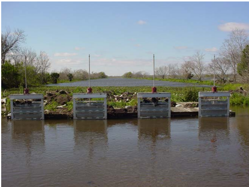
Photo #4 Site 26 The structure still has a small amount storm debris. The blockage of the culverts by storm debris has been cleared. The flow-meter, and all its attachments that were destroyed by the storm, will be replaced soon.
